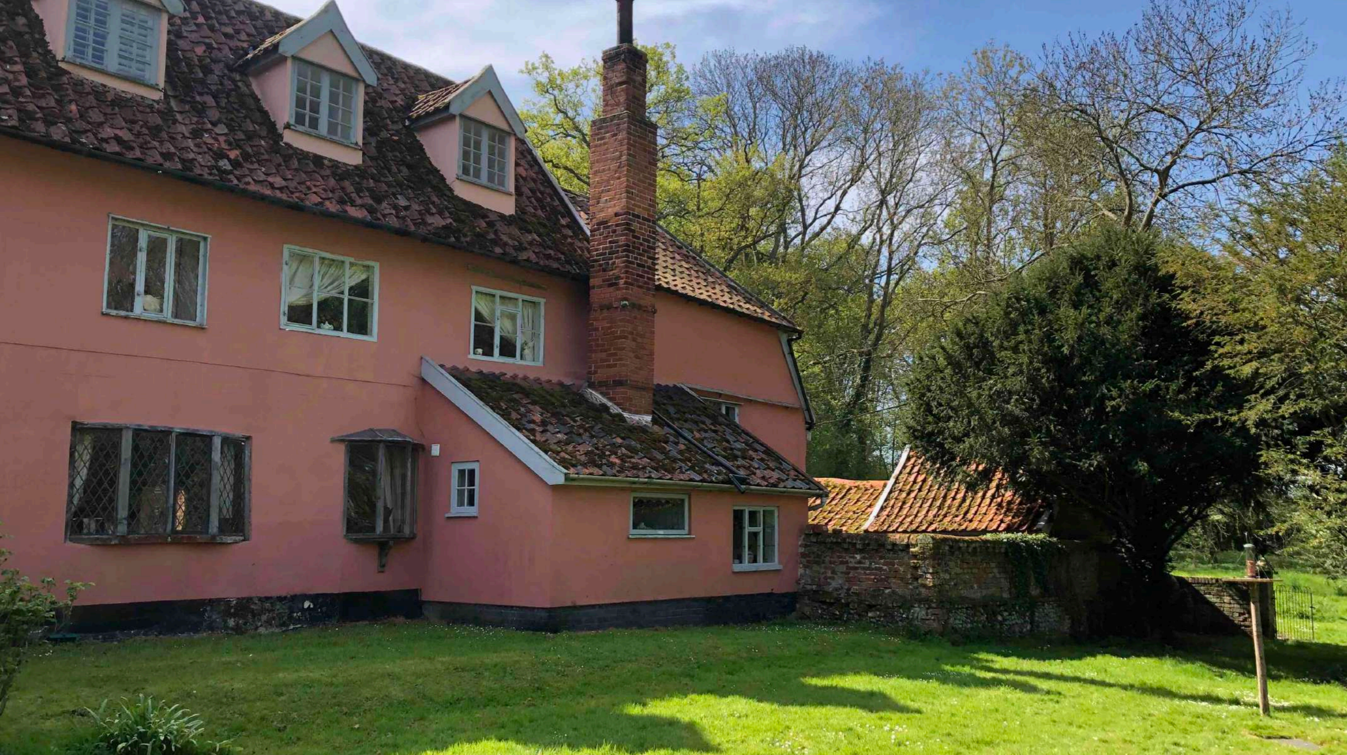
Rear view of Monks Hall showing 19th century and 20th century lean to and boiler house chimney proposed for removal
