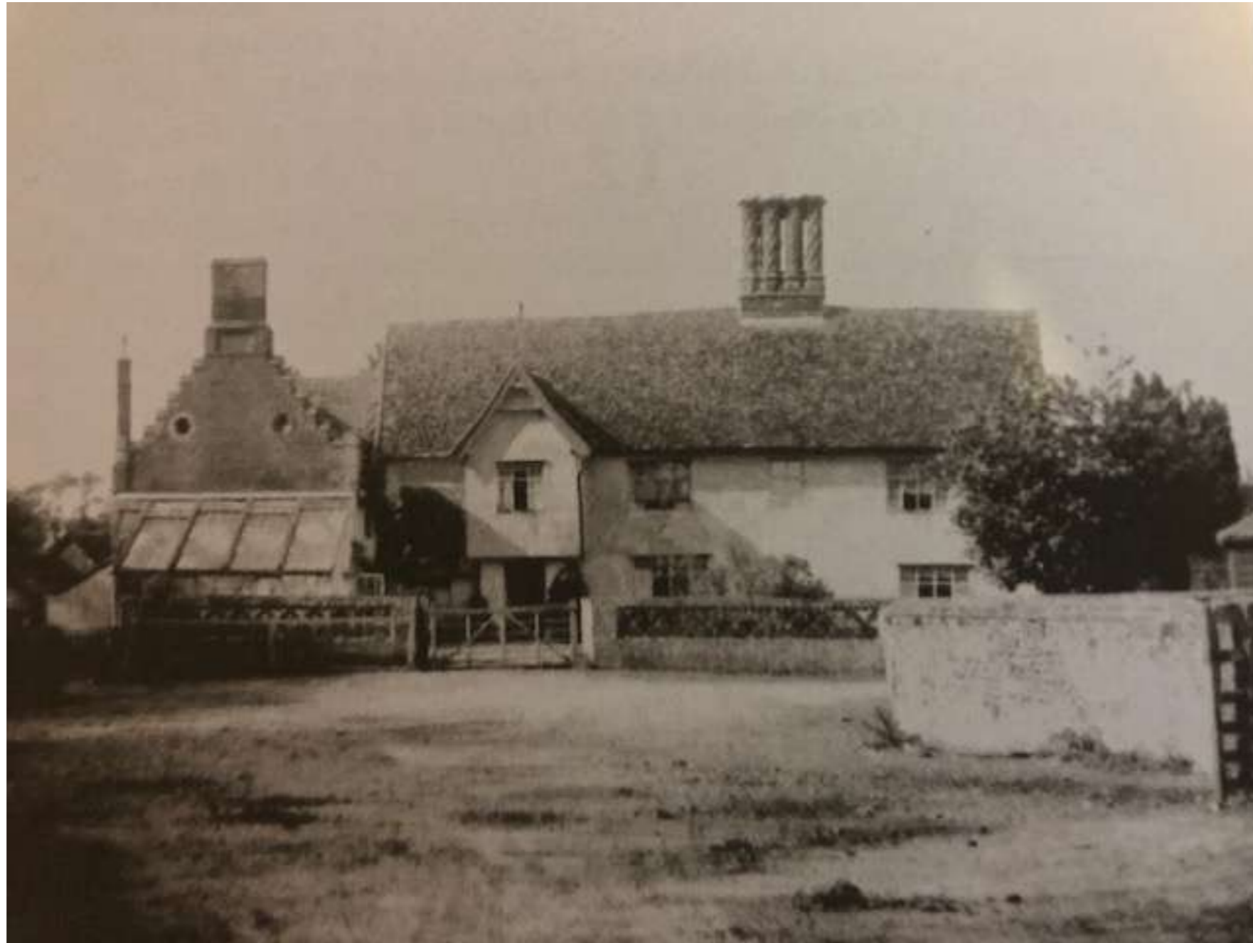
A late 19th century view of the house . Walls are rendered, a lean to Victorian greenhouse occupies the South gable and windows retain a more historical form. Extra windows inserted circa 1935 by Winn (Monks Hall - Elaine Murphy)
