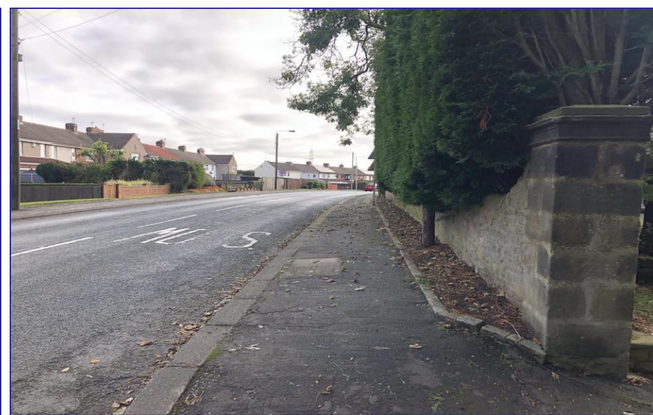
Photographic Plate 2 – A182 road at site entrance looking east.
