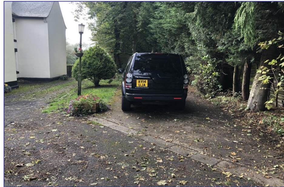
Photographic Plate 4 – Concrete hardstanding to side of Vicarage building that will provide access to new dwellings.
