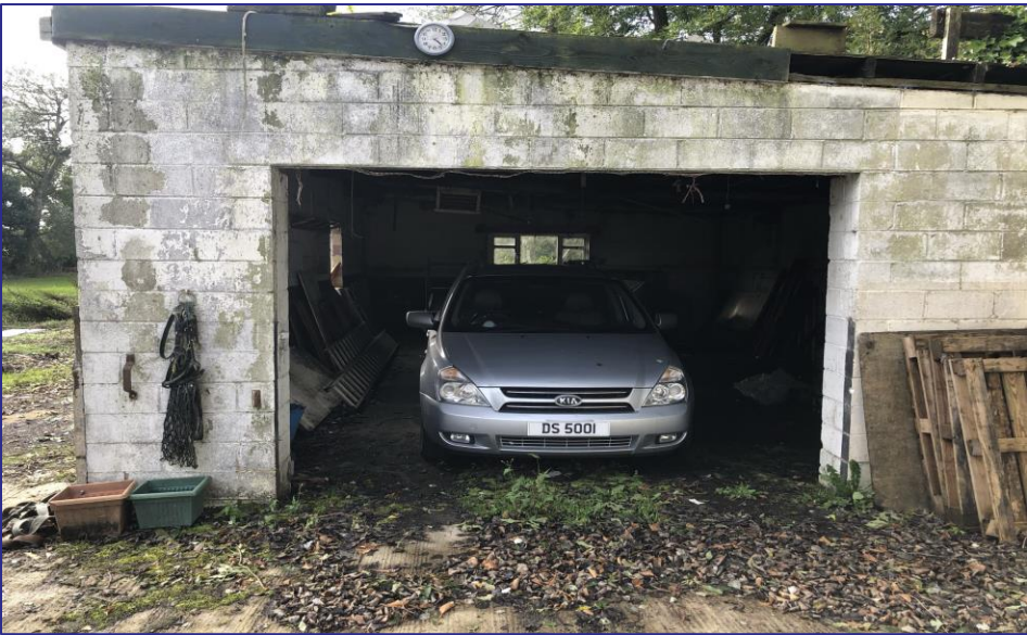
Photographic Plate 7 – Car in garage, also on concrete slab.
