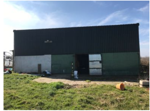
west elevation of barn
