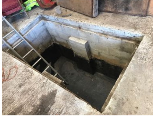
concrete lined inspection pit
