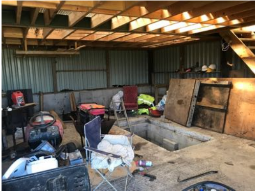
inside north area of barn
