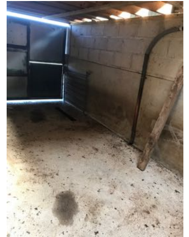
south section of barn
