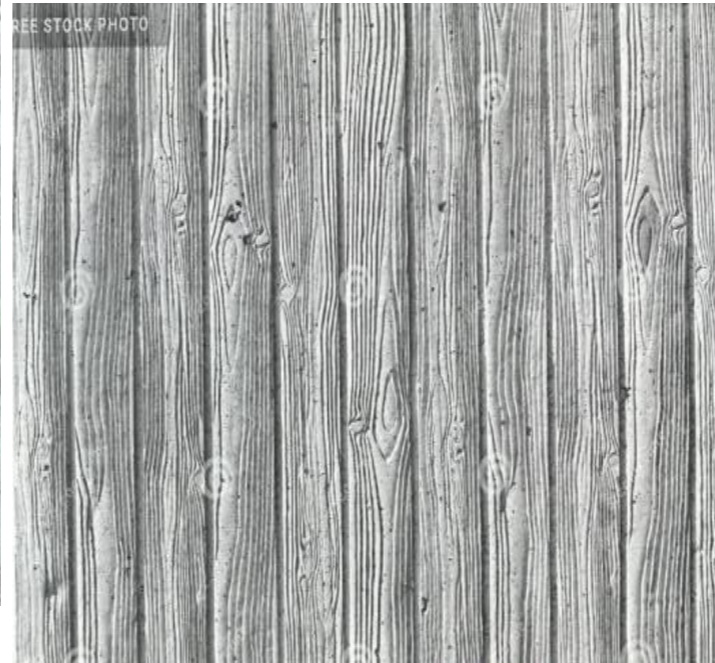
Pallet of Materials: Example of vertical timber cladding in concrete
