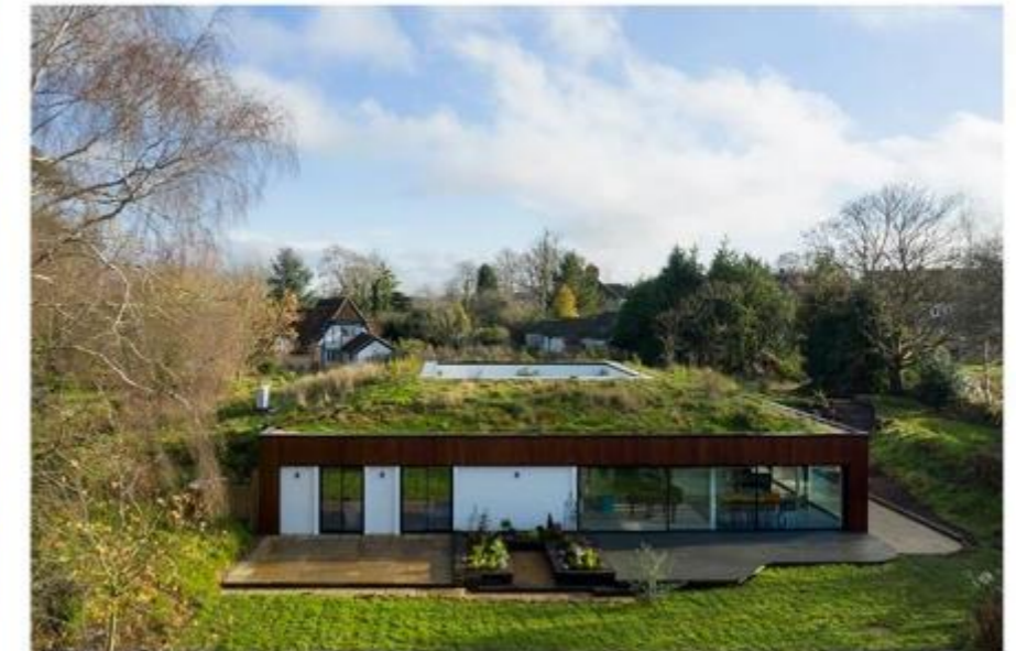
The timber cladding is western red cedar. Image: Jefferson Smith
