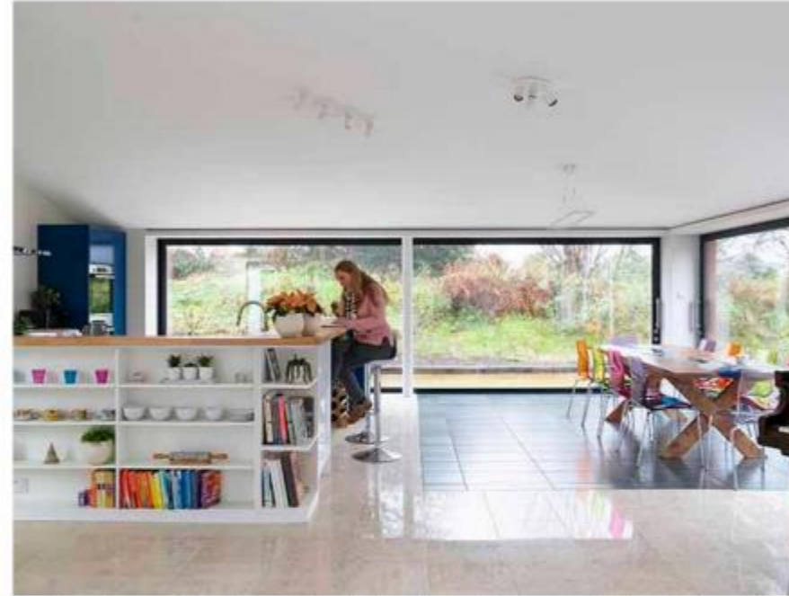
Black floor tiles absorb the sun's warmth, passing it to pipes to the hot water tank. Photo: Jefferson Smith
