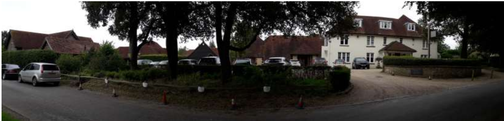
Panoramic street elevation (existing laundry to be extended on left hand side)
