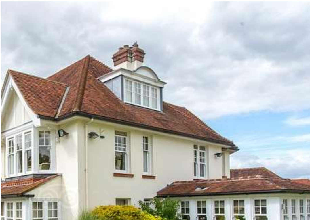
Photograph No. 06 – View of section 2 of B01, window proposed for new balcony
