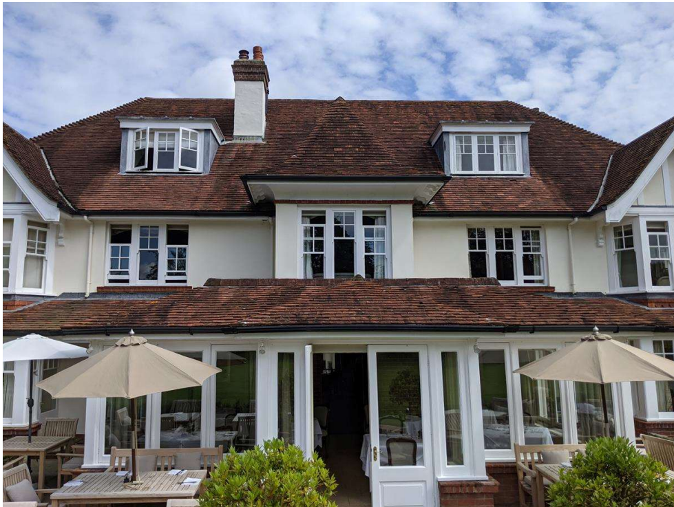
Photograph No. 02 – View of Section 1 of B01, a day roost of 8no. common pipistrelles inhabit this roof area.
