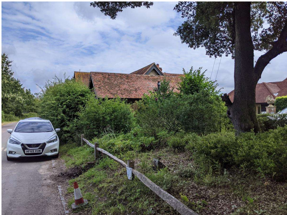
Photograph No. 10 – View towards B02 from the south showing the introduced shrubs proposed for removal to accommodate an extension.
