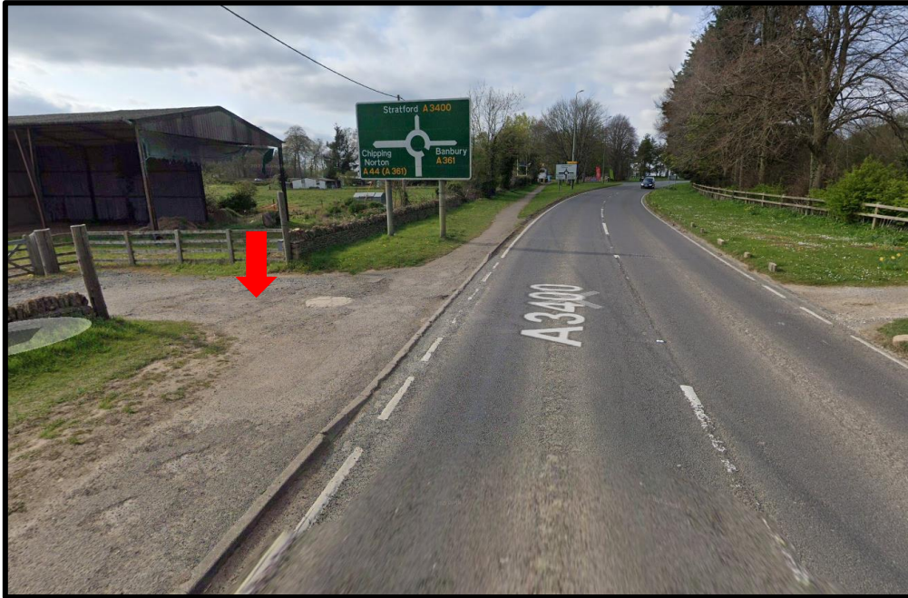
Figure 3.2 – View to North of Existing Site Access
