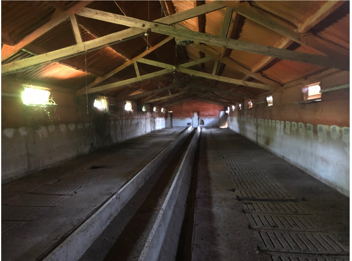
Picture 4 – Internal view of Barn B
