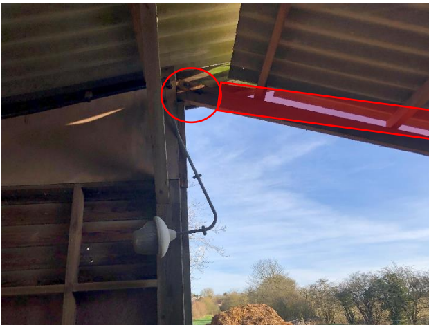
Photos 3 & 4: South eastern corner of Building 4, showing split in wooden structural beams
