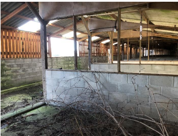
Photo 7: Internal view of Building 4, southern section
