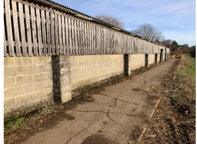
Photo 6: Southern elevation of Building 4, with adjoining concrete
