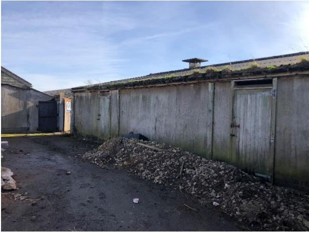
Photo 3: Northern elevation of Building 3
