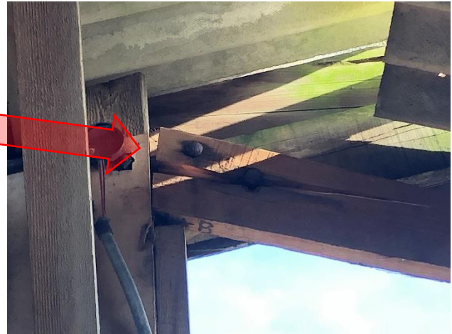
Photos 3 & 4: South eastern corner of Building 4, showing split in wooden structural beams
