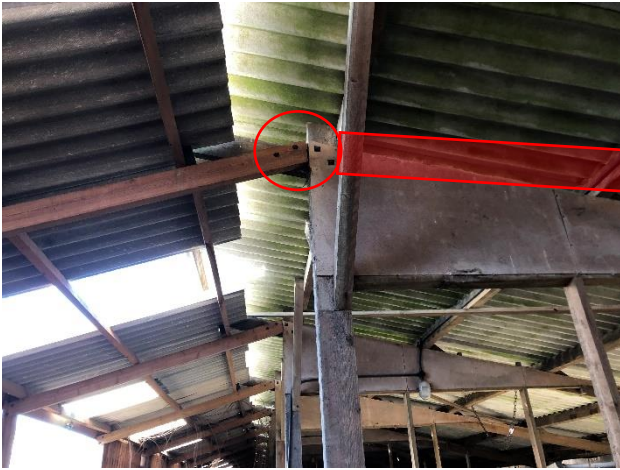
Photos 1 & 2: Southern section of Building 4, showing small gap between wooden structural beams. A number of these are present along the southern length of Building 4
