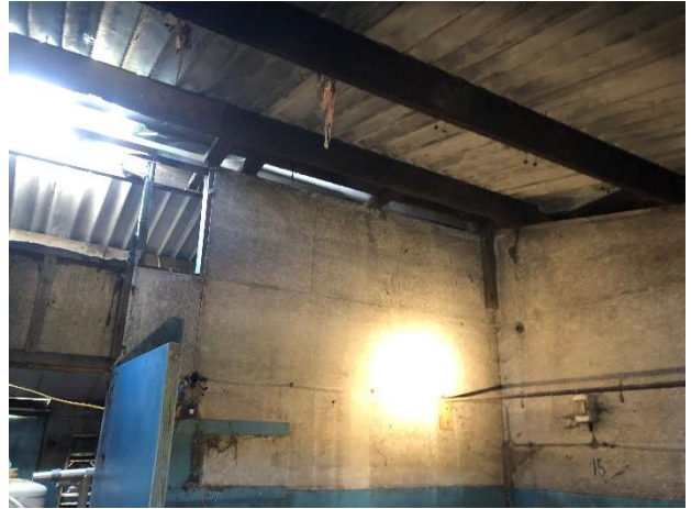
Photo 4: Internal view of Building 3
