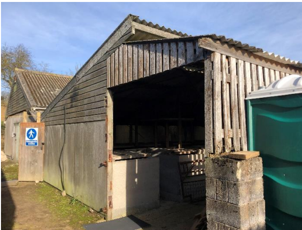
Photo 5: Western elevations of Building 4, showing the two adjoining sections
