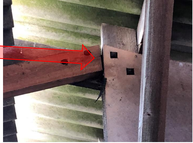
Photos 1 & 2: Southern section of Building 4, showing small gap between wooden structural beams. A number of these are present along the southern length of Building 4
