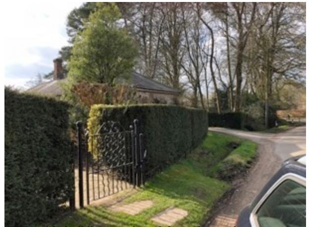
4 The stable building as viewed from the road, looking north.
