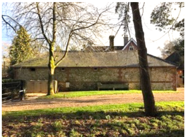
6 North-west (rear) elevation. It is planned to build an oak framed shelter against the central part of this elevation.
