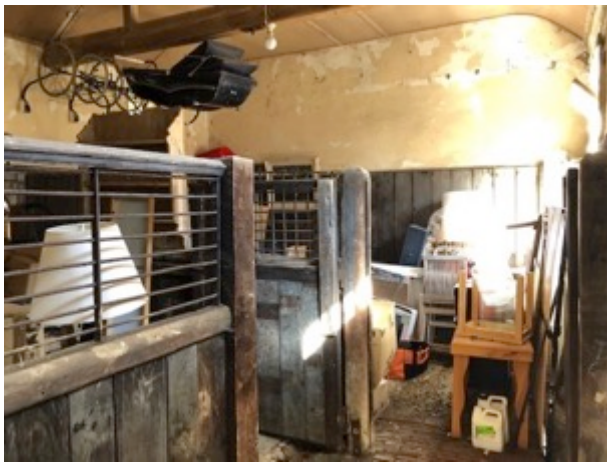
9 Main room, showing the loose box divisions and boarding to the walls.
