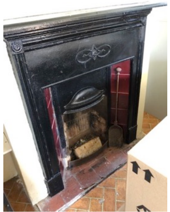
8 Early C20 cast iron fire grate and surround in the former tack room.
