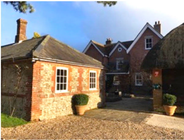
3 Looking towards the main house, showing the extended elevation of c. 2001. The two windows in the stable building were inserted at about the same time.
