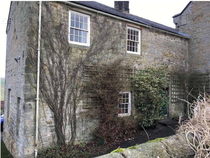
Photo 10 North wing south elevation from behind garden wall.
