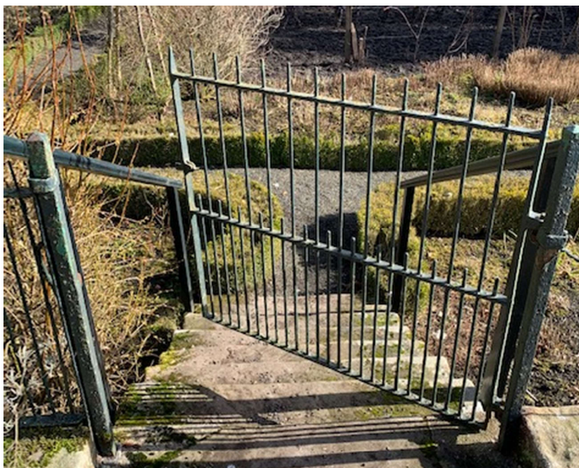
Photo 13 Existing gate to east walled garden.
