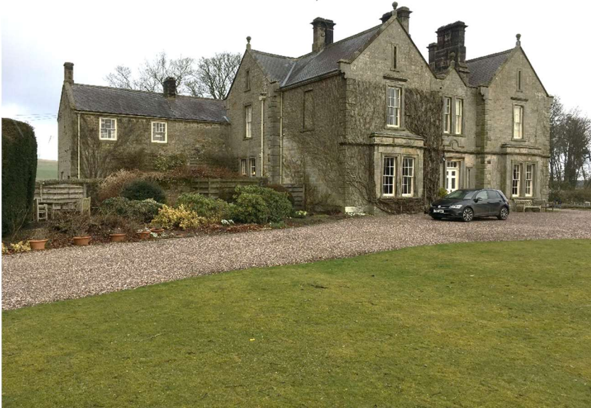
Photo 1 – cover: View of Carrycoats Hall from the south
