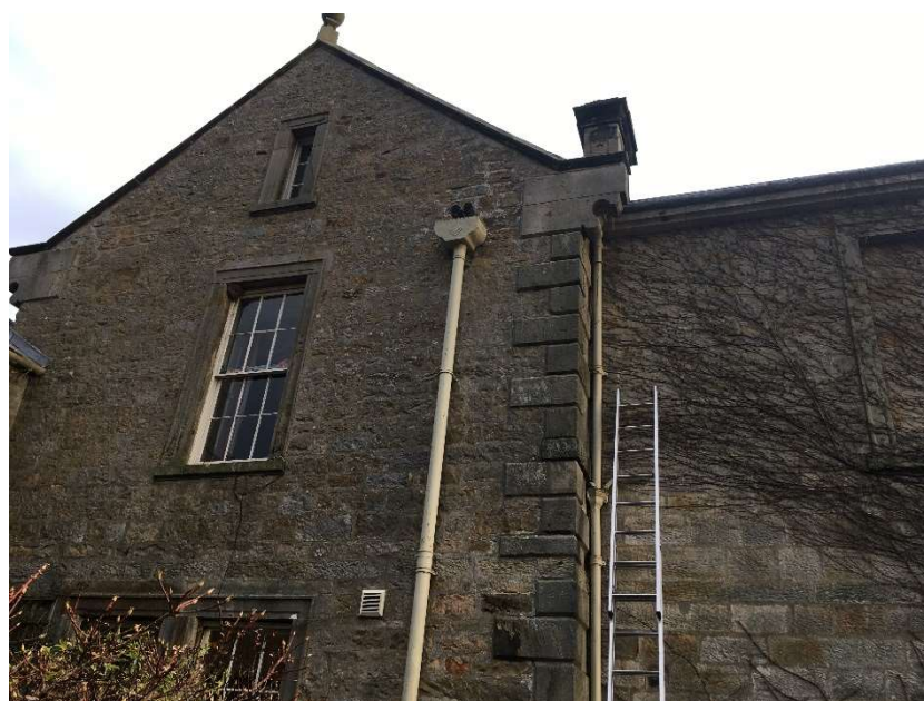
Photo 5 Close up of west gable showing kneeler stones.
