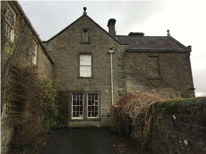
Photo 8 West gable from west.
