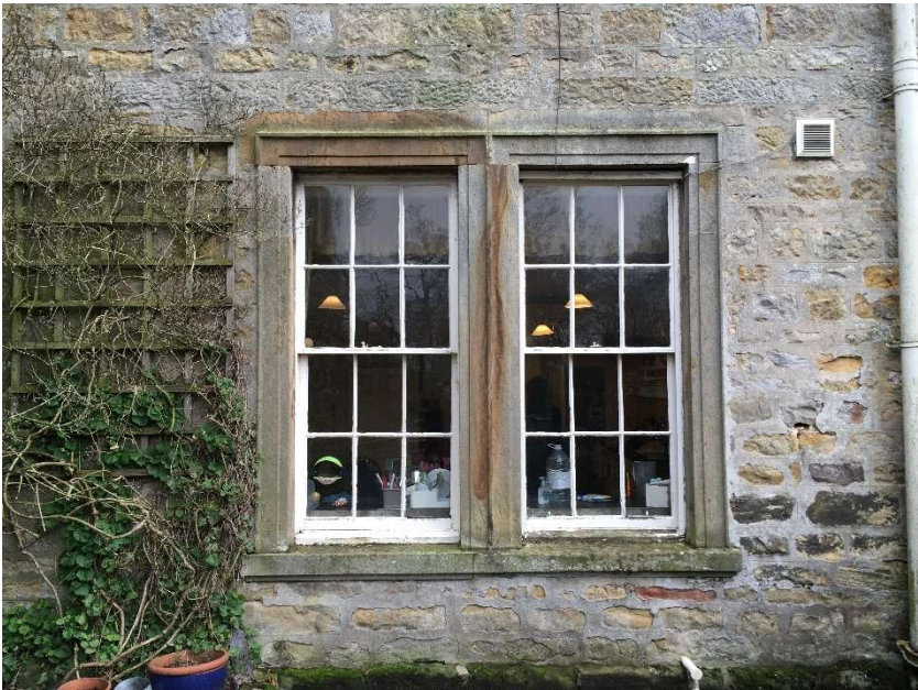
Photo 9 Close up of kitchen window
