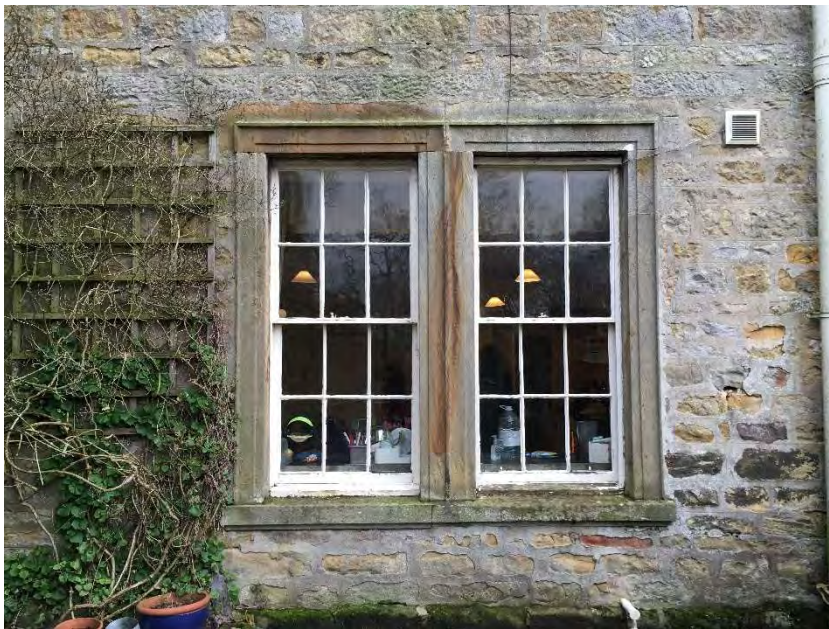
Photo 9 Close up of kitchen window
