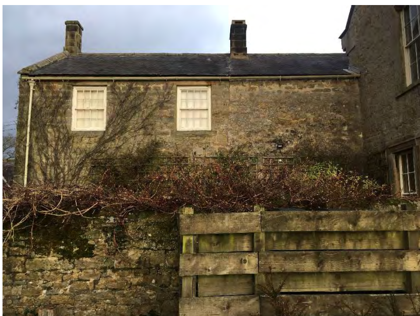
Photo 7 North Wing from south with oil tank screen and garden wall in foreground.
