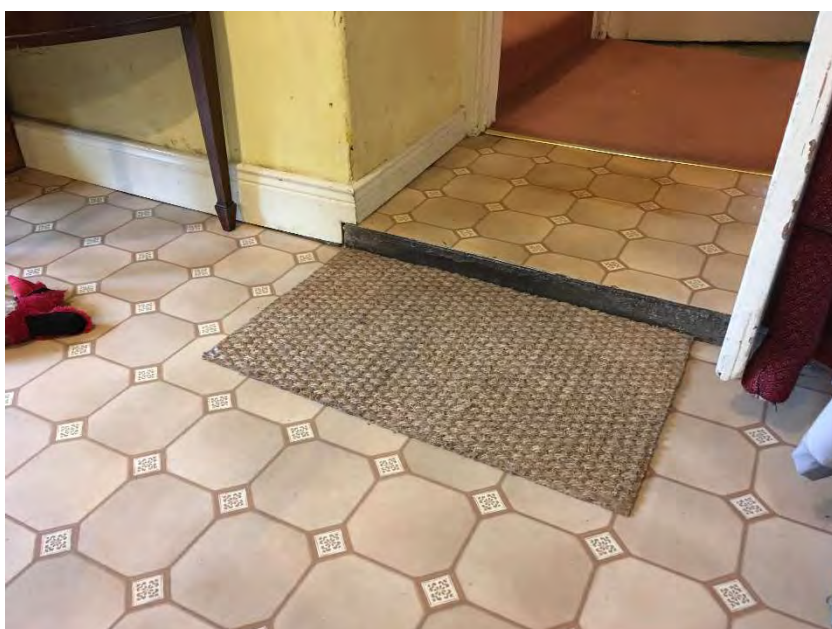
Photo 12 Vinyl flooring to kitchen over cement screed with 70mm step up into north wing.
