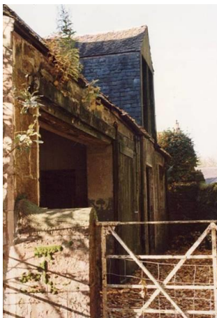
Building 1988 prior conversion
