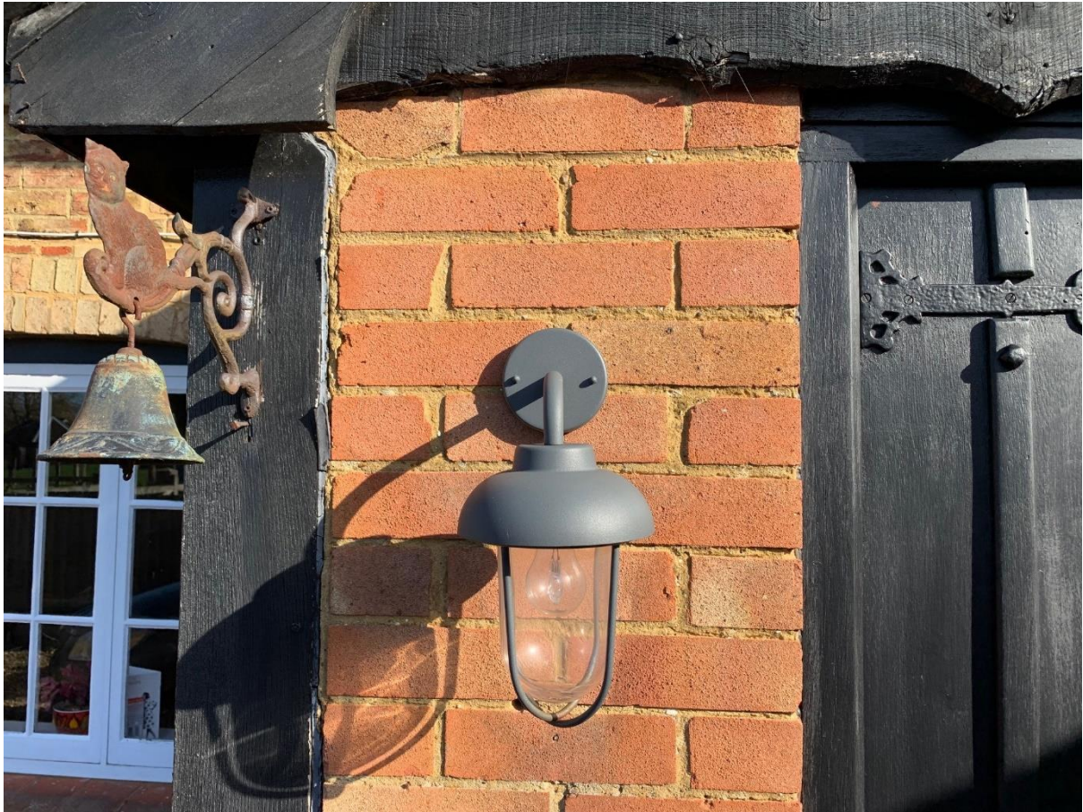
Bricks as existing to front elevation to main house
