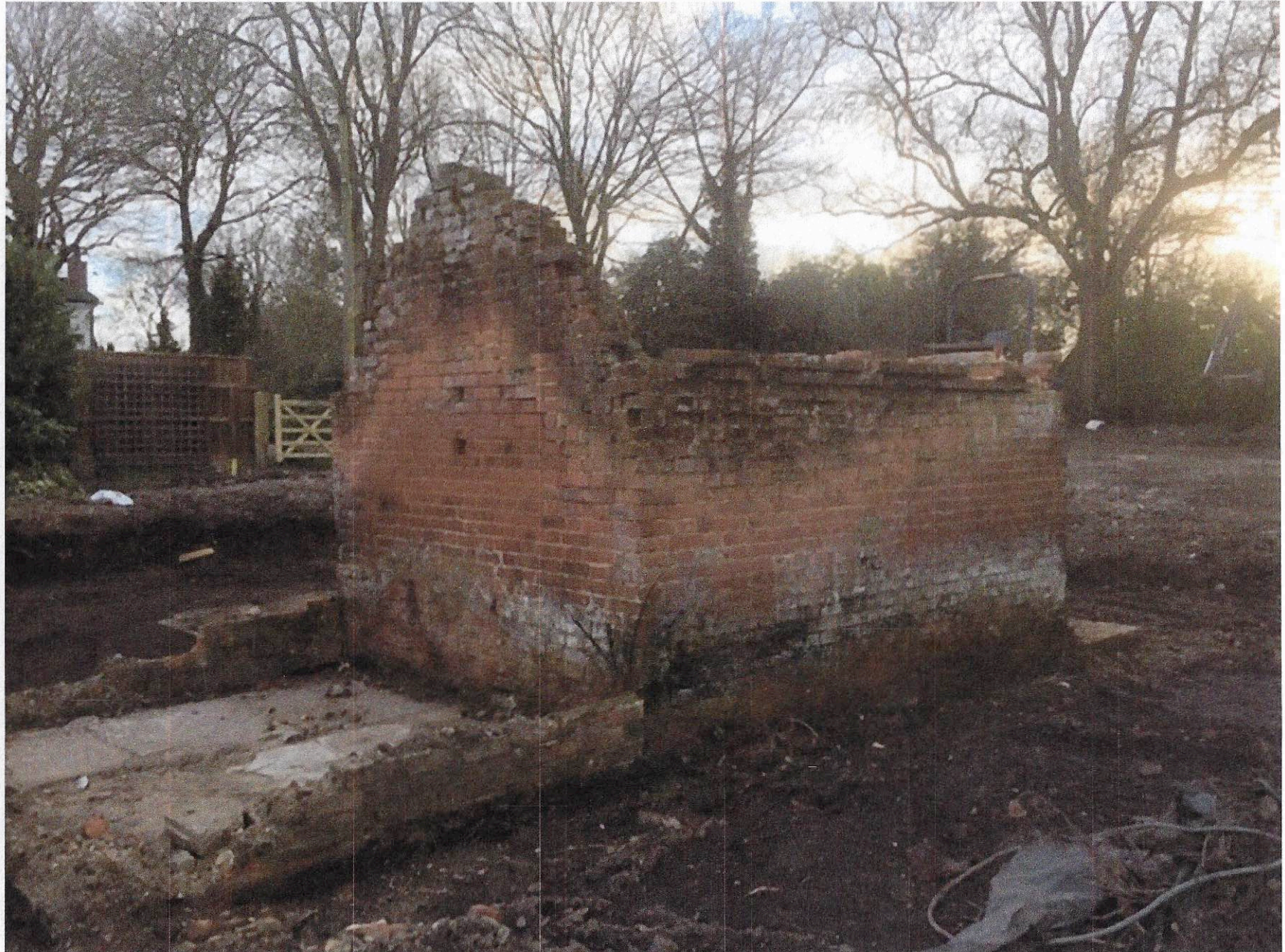
PHOTO - previous structure
