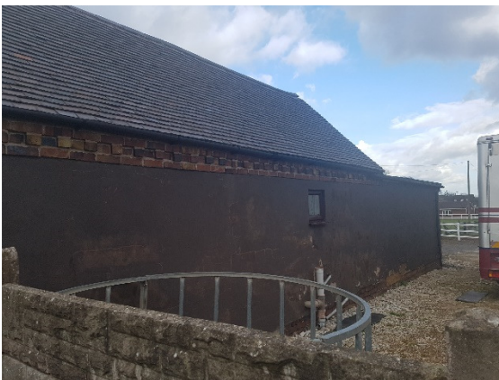
E: Part Side View of Existing Stable Unit
