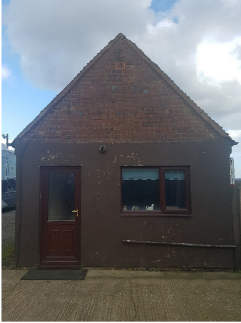
C: Front Entrance to Existing Stable Unit
