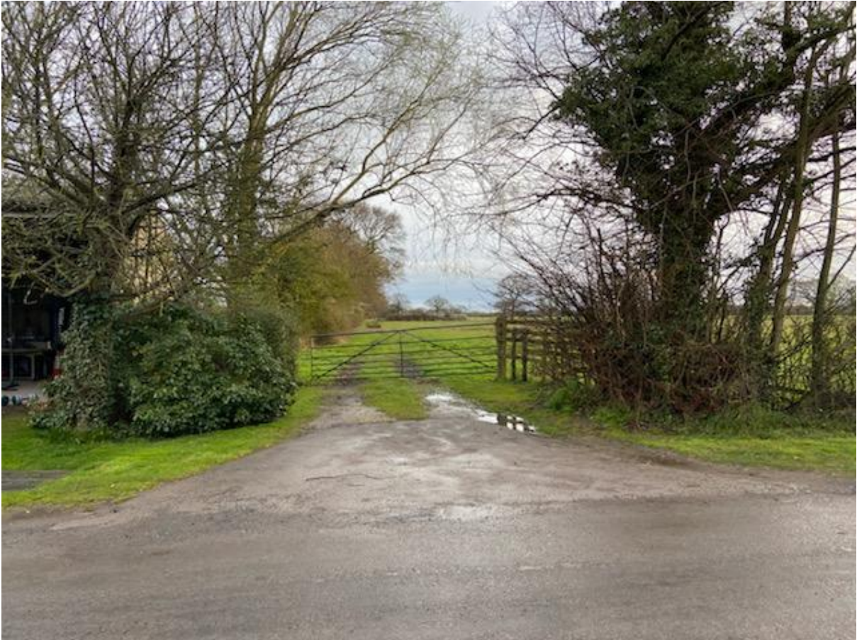
Current gateway into field to west of Laytham Road from existing access track. 3m wide gate: low branches of trees overhanging gateway. Large farm vehicles cannot turn from access track (2.5m wide at this point) into the field.
