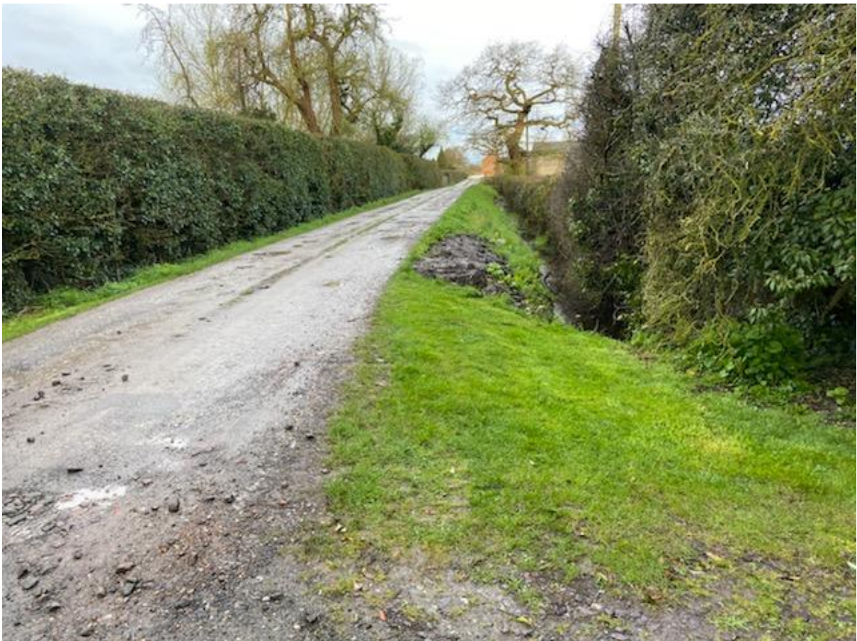
Western section of existing access track 2.5m wide: dropped verges, hedges and ditch.
