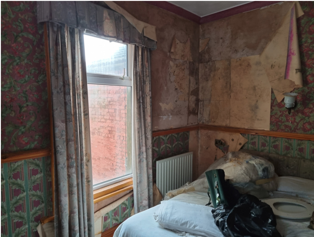
Existing First Floor Bedroom
