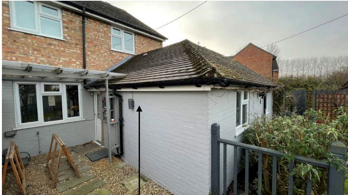
Single storey extension proposed to be attached to the existing wall shown here for the new kitchen dinner.
