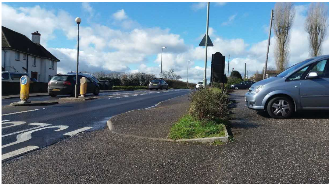
Photograph 3 – The existing access looking right on egress.
