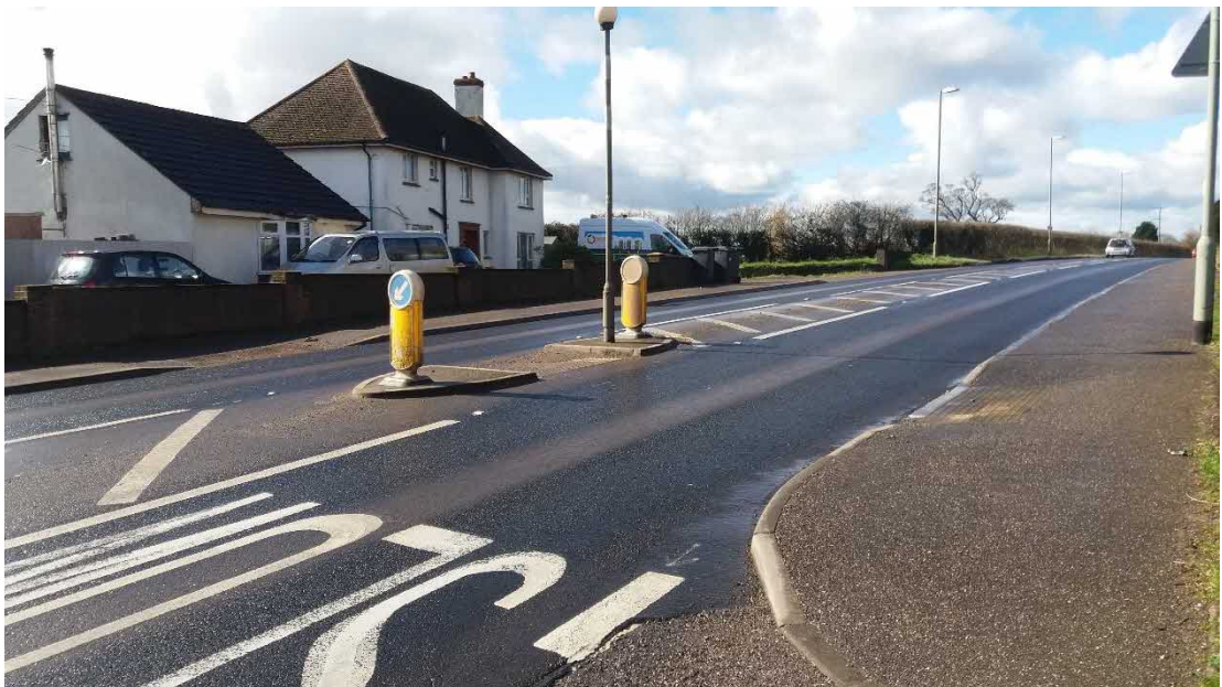
Photograph 5 – The A3052 pedestrian refuge just west of the application site access.
