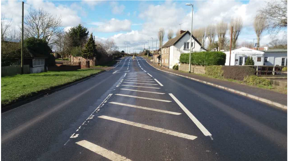
Photograph 4 – The A3052 right turn ghost island into the application site looking west.
