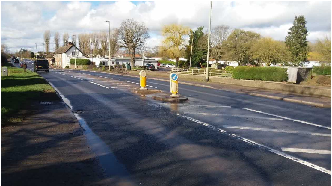
Photograph 6 – The A3052 looking west towards the application site showing the pedestrian refuge.
