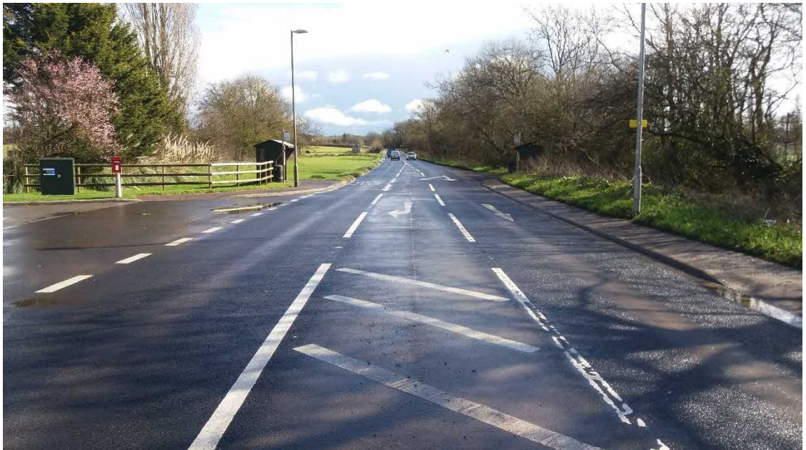
Photograph 7 – The A3052 looking east beyond the application site showing the bus stops.
