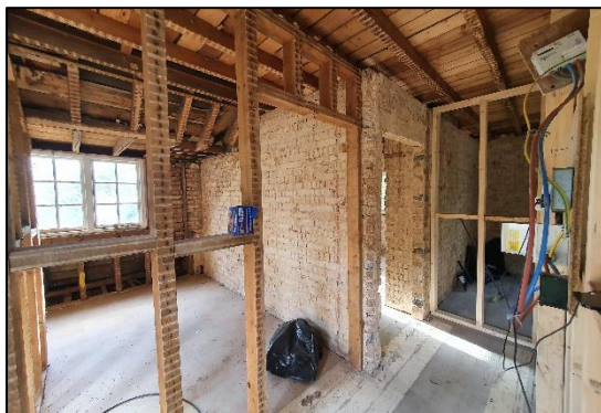
Figure 6: Holme House – internal view
