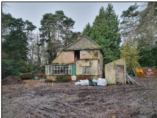
Figure 1: Cleared ground around the house, with mature trees to eastern boundary.
