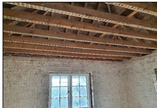
Figure 7: Holme House – internal view.
