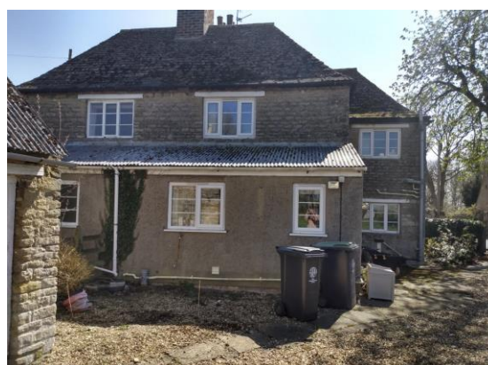
View of existing rear extension
