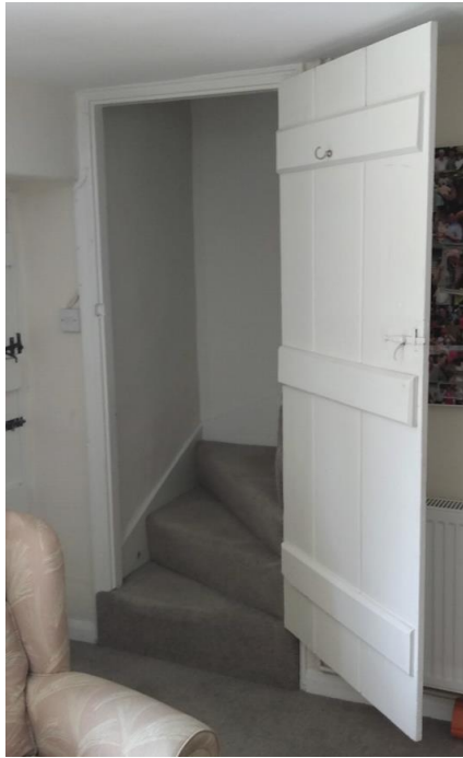
View of existing stairs at ground floor
