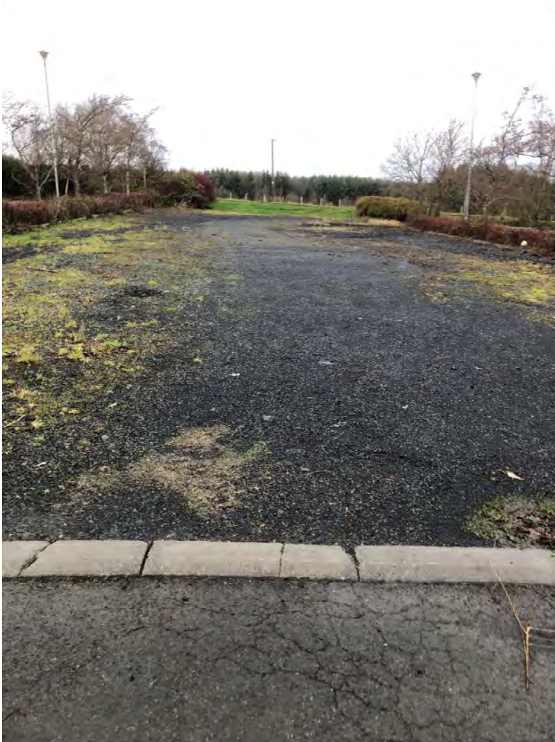
11. Centre of site looking north across gravel car park
