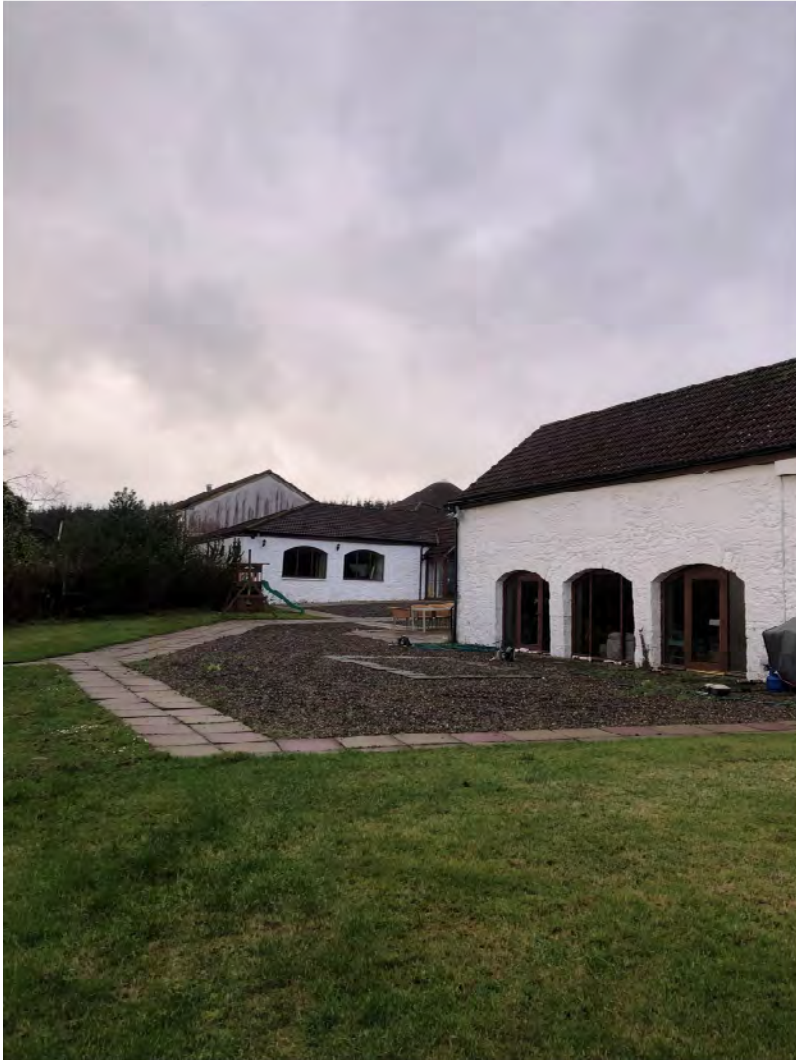
15. SE (offsite) of site looking west
