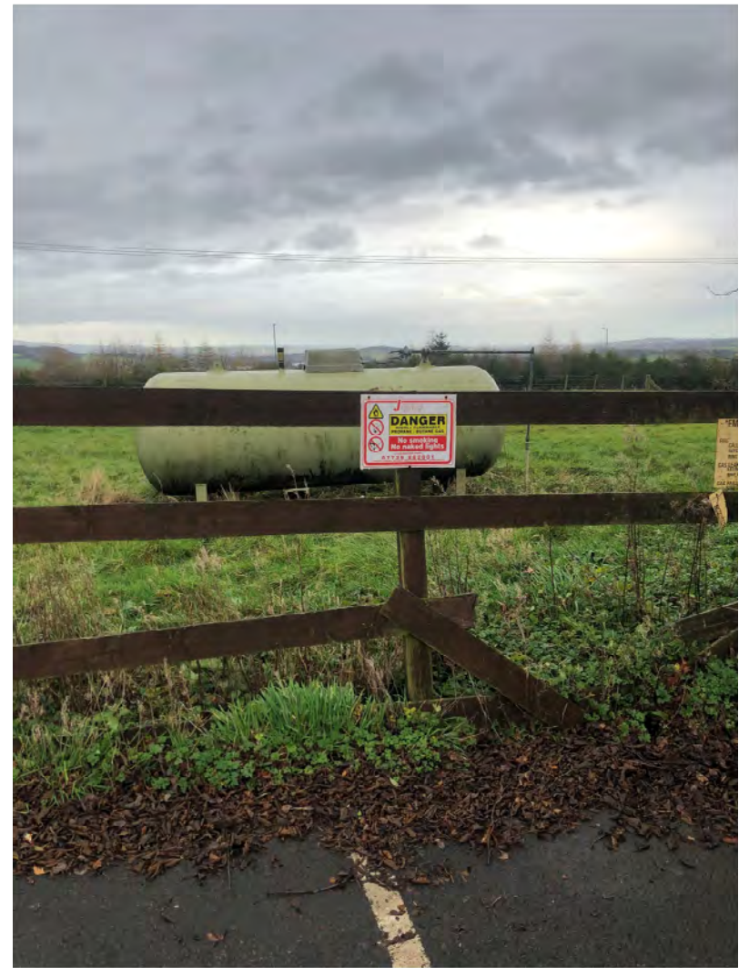
12. Centre of site looking east at propane tank
