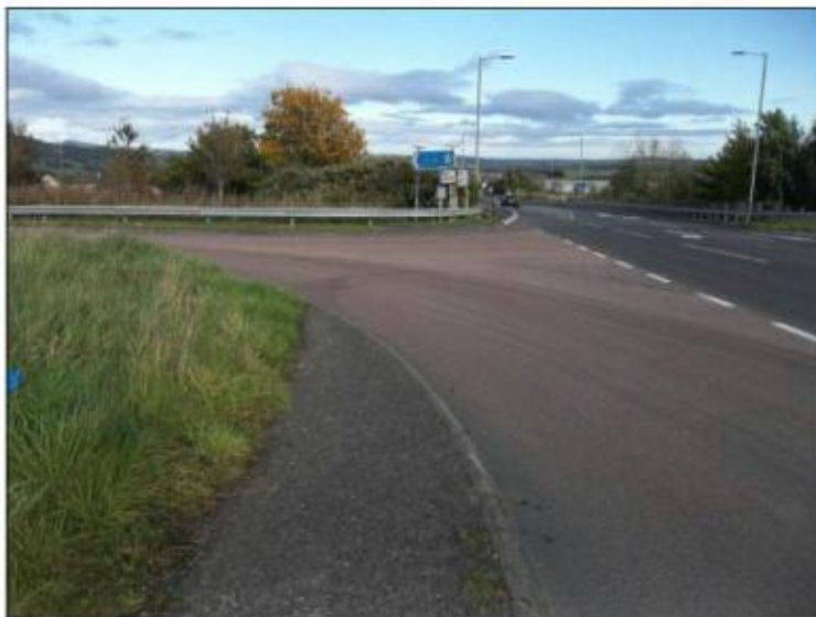
Photo 2.10 – Northern footway from the B914 looking eastwards across the M90 southbound off slip
