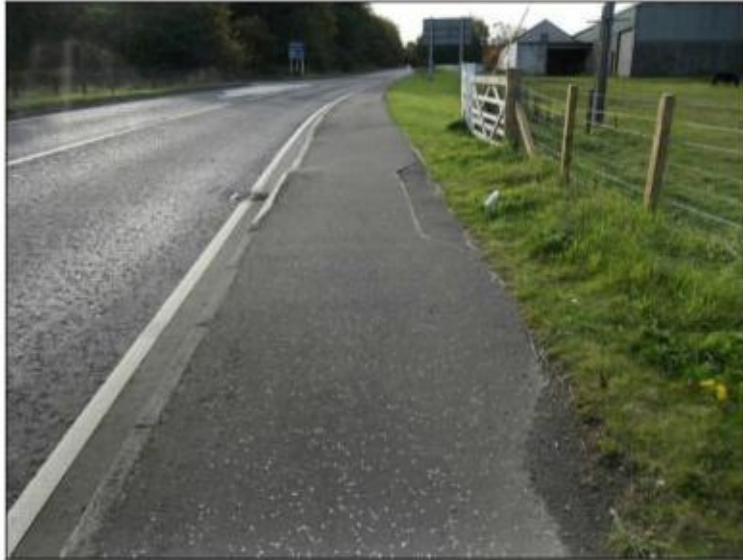
Photo 2.3 – Northern footway along the B914 looking westwards from the site access
