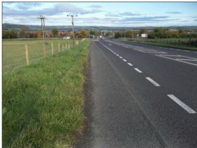
Photo 2.8 – Northern footway along the B914 looking eastwards from the site access towards the M90 Junction 4 interchange
