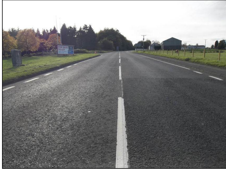
Photo 2.31 – B914 looking west towards the existing site access
