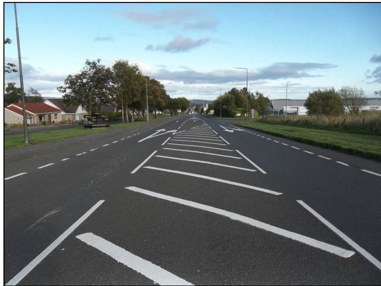
Photo 2.38 – A909 Cocklaw Street looking eastwards from the M90 Junction 4 interchange
