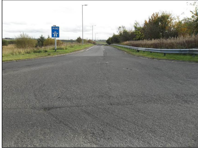
Photo 2.37 – M90 Junction 4 southbound on slip
