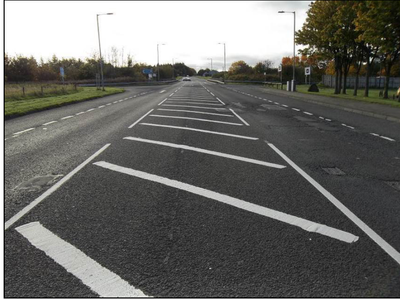
Photo 2.39 – A909 Cocklaw Street looking westwards towards the M90 Junction 4 interchange
