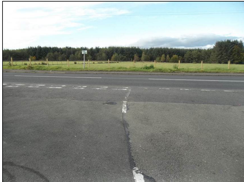
Photo 2.26 – Site access looking towards the B914
