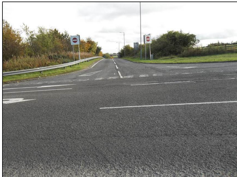
Photo 2.34 – M90 Junction 4 northbound off slip
