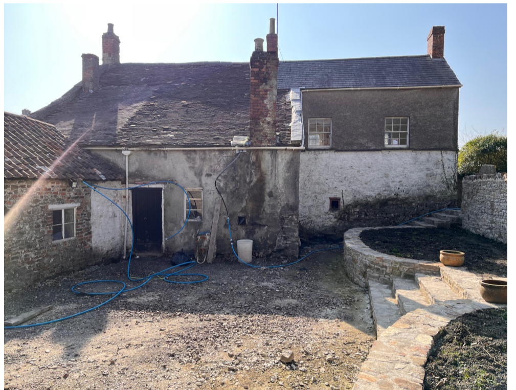
3. North elevation of the main farm house
