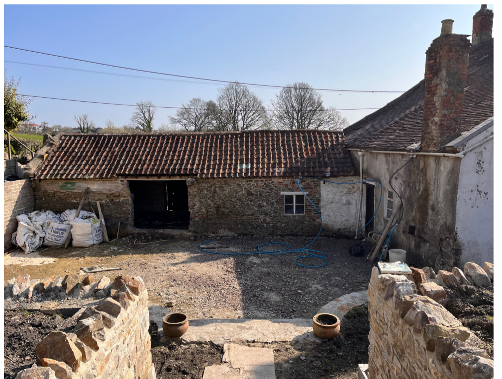
4. West elevation of the barn
