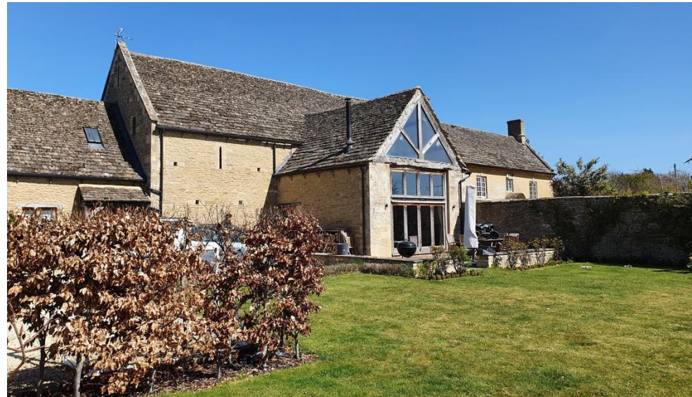
Photograph A: View of Priory Barn and Park House in background.
