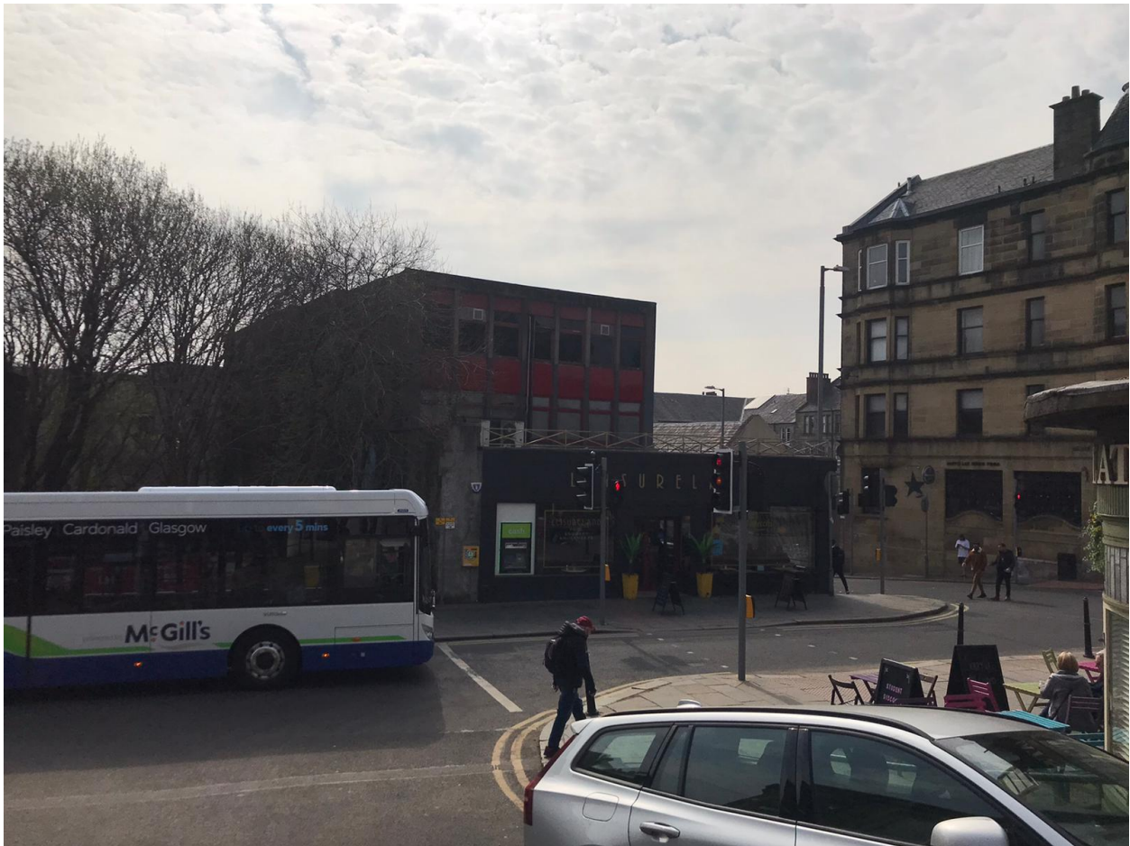
Figure 2: Pedestrian Crossing on High Street
