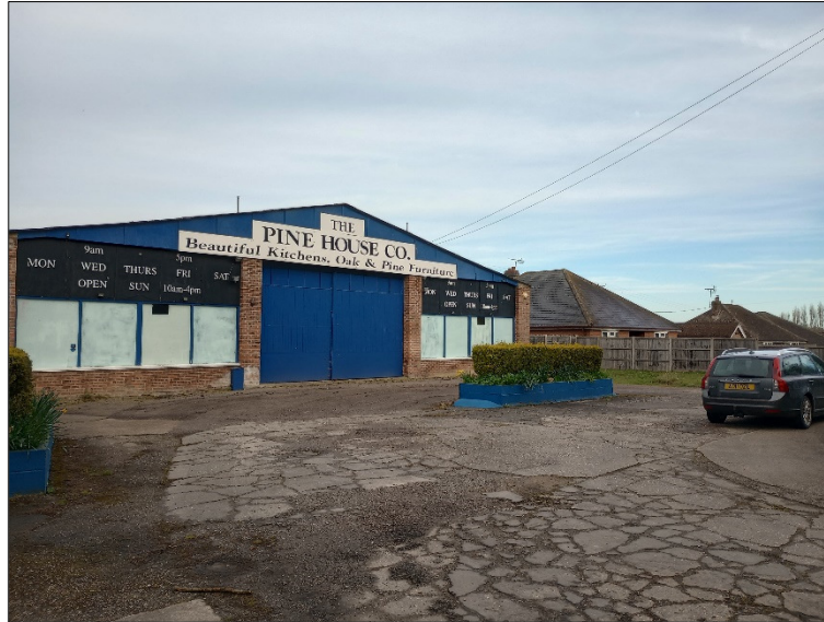
Figure 2.3: View of front elevation of the building
