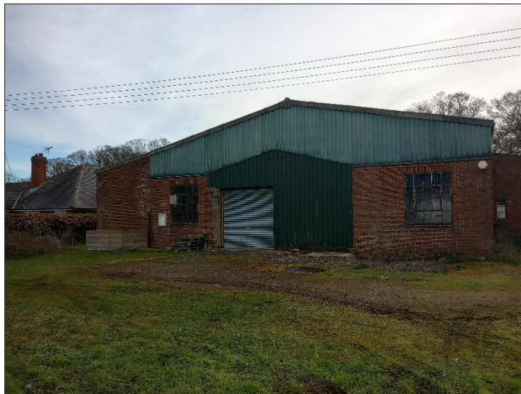
Figure 2.4: View of rear elevation of the building
