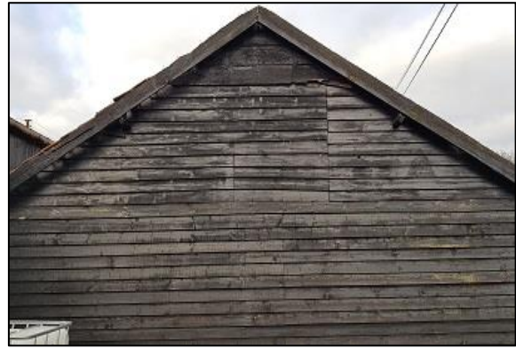
Figure 6: Building 2 – cladded gable end.
