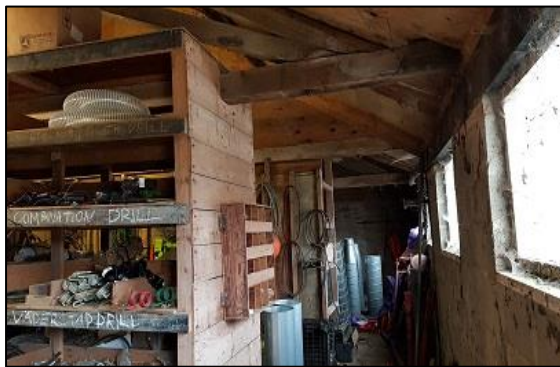
Figure 7: Building 2 – interior view.
