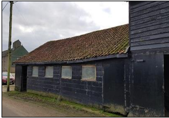
Figure 5: Building 2 – northern aspect.
