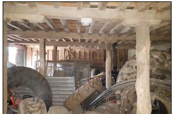
Figure 9: Building 3 – Ground floor interior.
