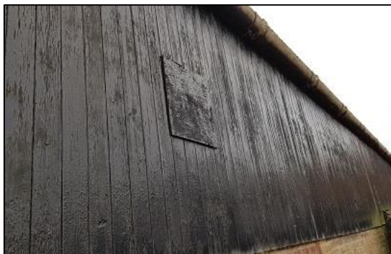
Figure 3: Tightly sealed vertical cladding.
