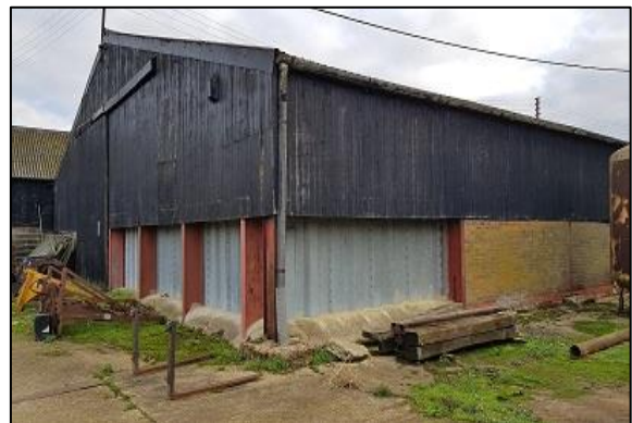
Figure 2: Building 1 – north-western aspects.
