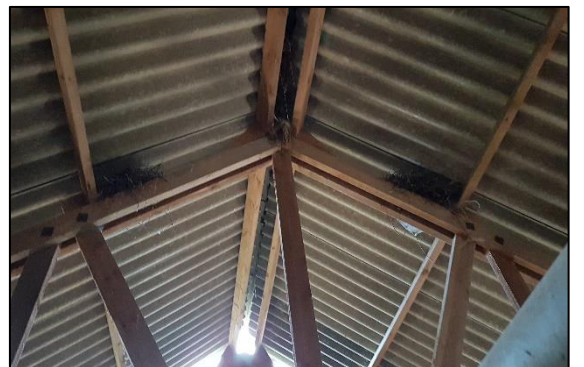
Figure 11: Building 3 – unlined corrugated roof with narrow beams.
