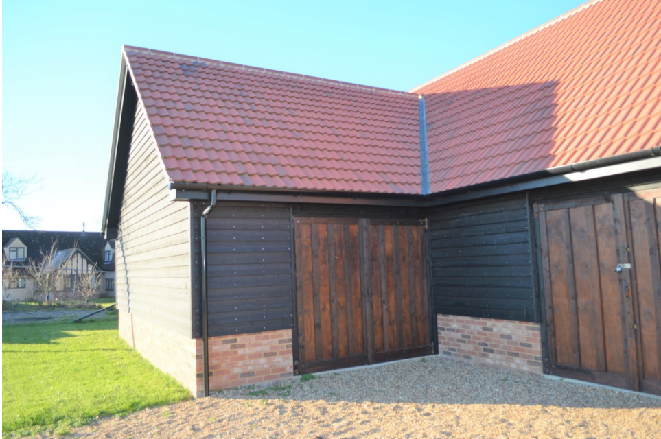
Photo 2 – Workshop Doors. Note well fitted external finishes.
