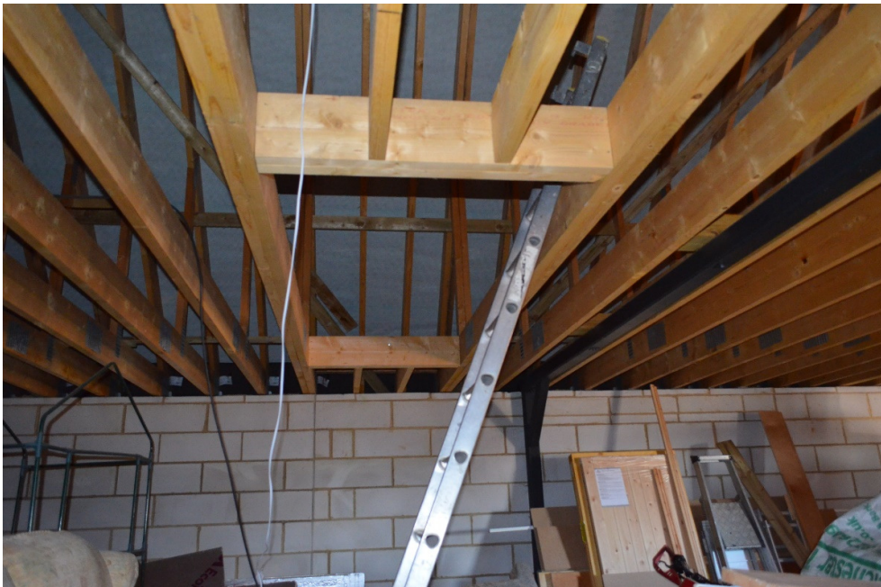
Photo 3 – Internal View – Note modern roof trusses, breathable felt & block external walling.
