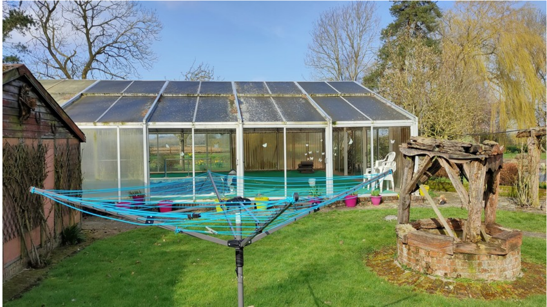
Courtyard view. RH section of pool removed. Building to LH to be clad in weatherboarding
