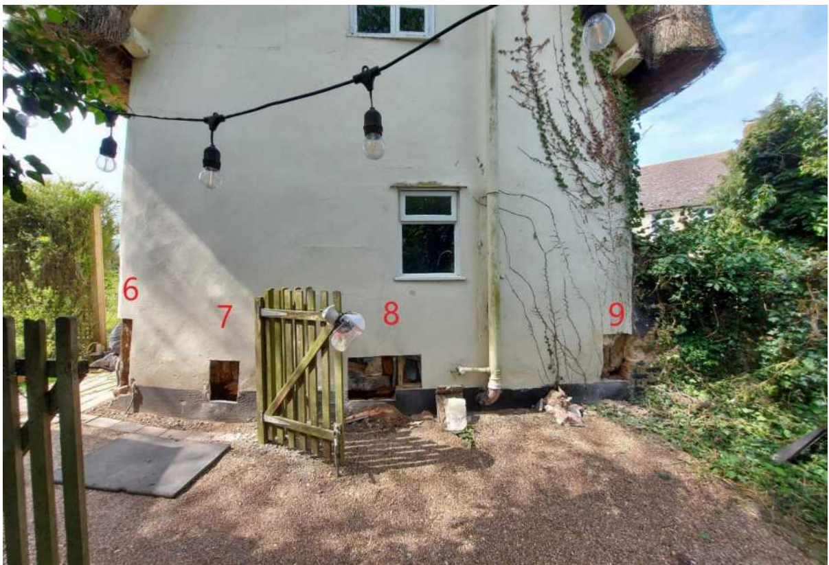
Below, the east elevation with four sections of render removed.
