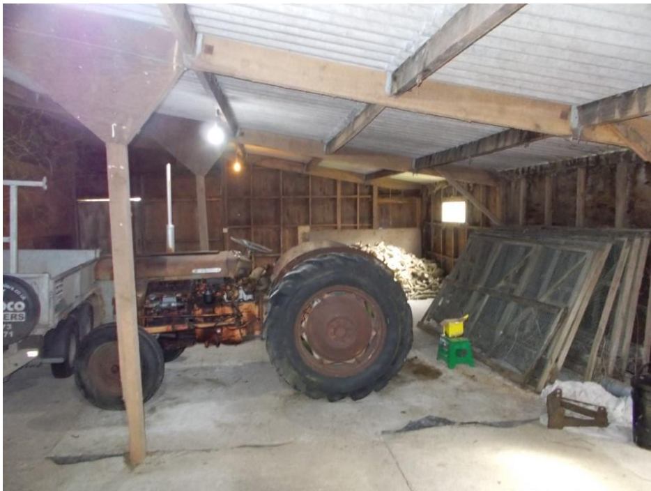
Photo 6 – Principal rafter and purlins
