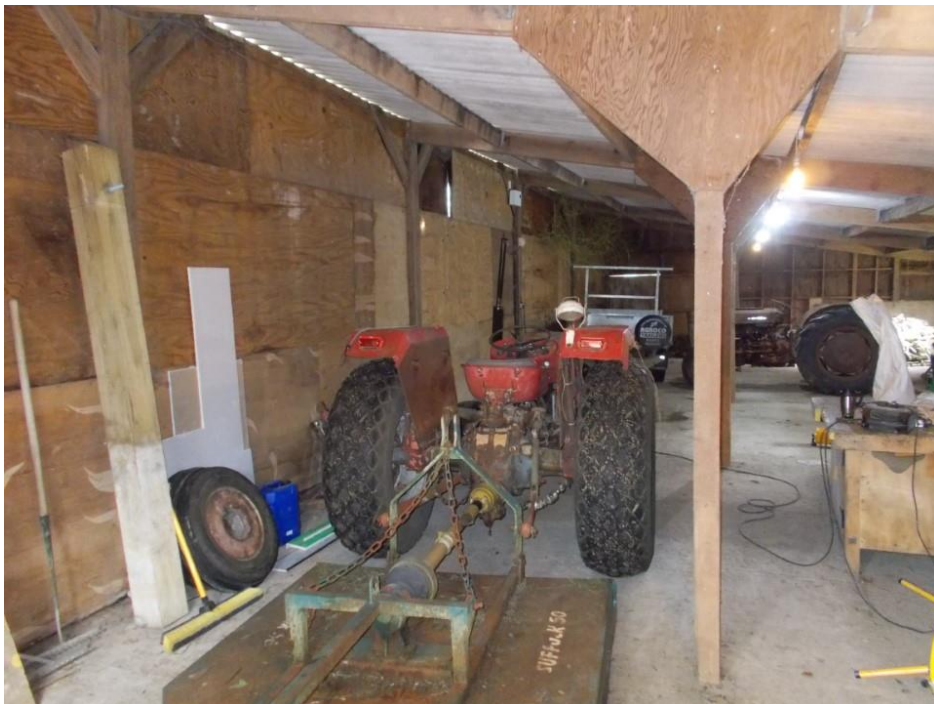
Photo 4 – Interior – intermediate post support
