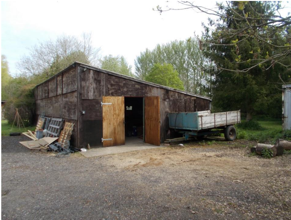
Photo 1 – South Gable End
