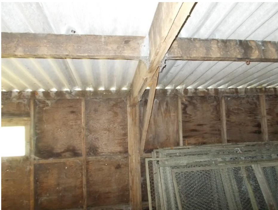
Photo 8 – Principal rafter, external post and wall panel detail
