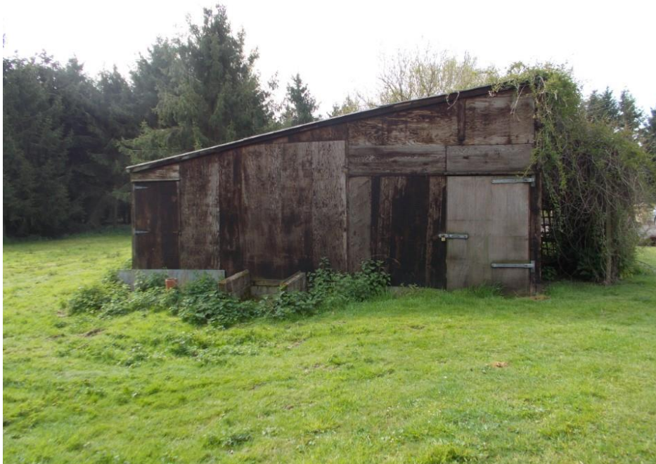
Photo 2 – North Gable End
