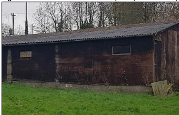
Figure 3: The barn and roof – eastern aspect.
