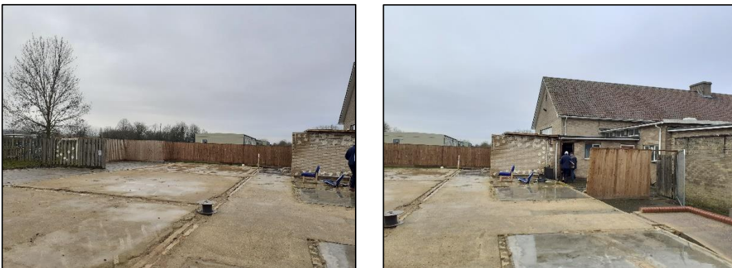
Figure 7 & 8: Fire Damaged School previously demolished
