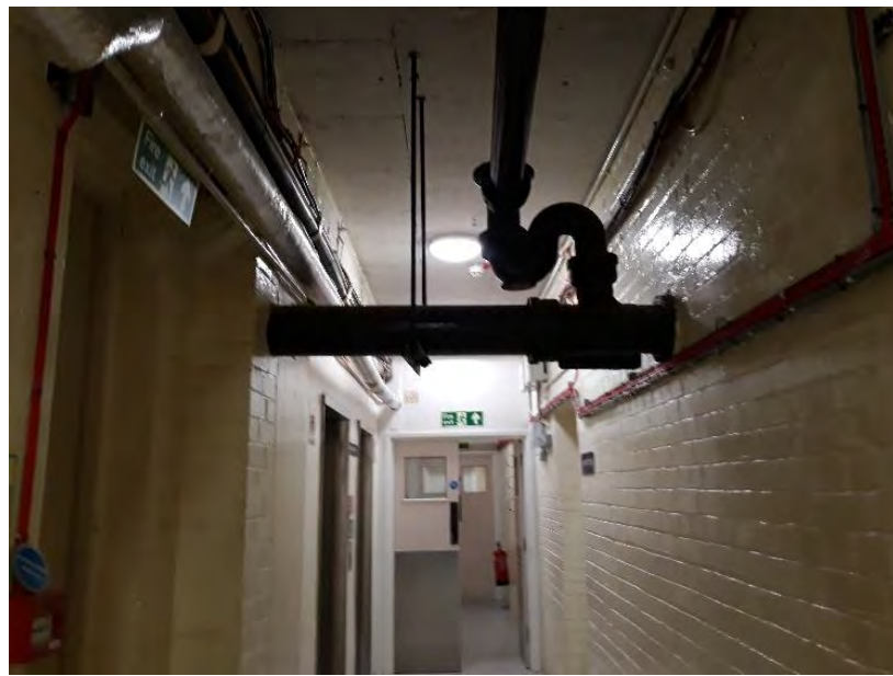
Figure 8.3.3 Typical combined drain outfall to external drainage
