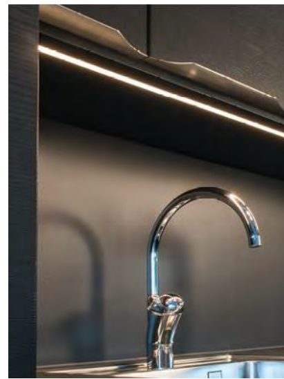
Figure 9.7.6 Typical example of LED tape for the kitchens.
