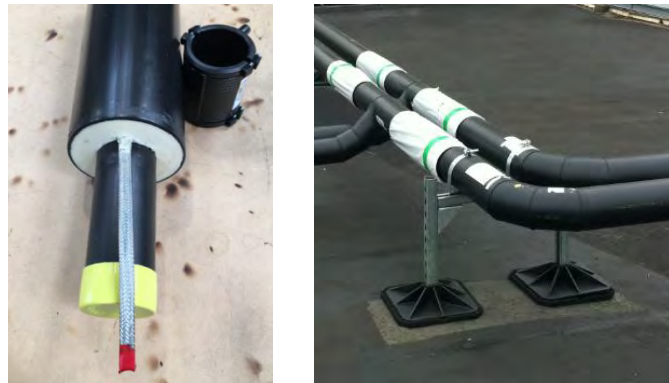
Figure 8.10.2 Typical frost protected, external water distribution pipework
