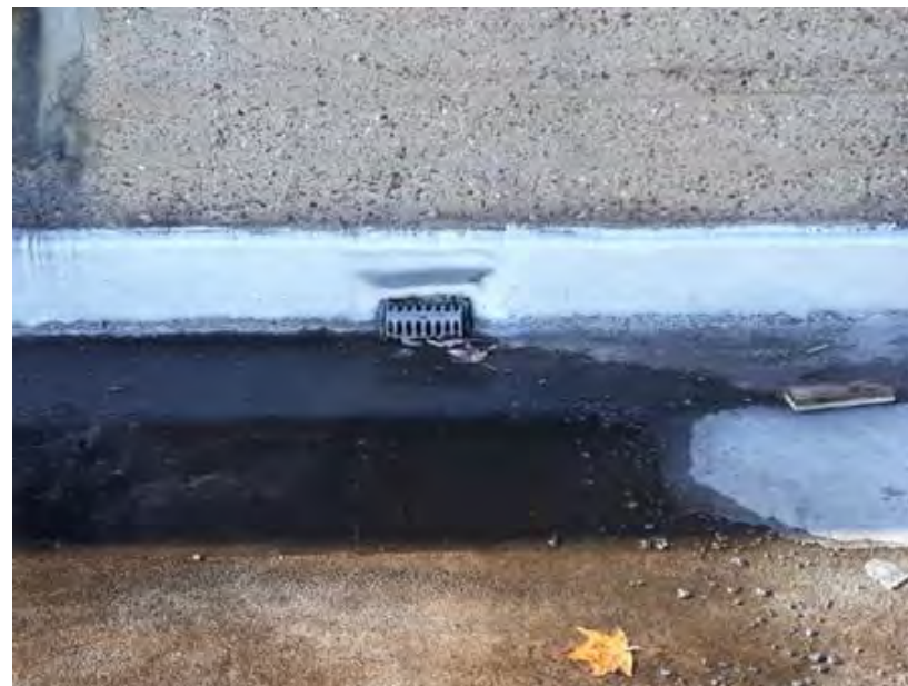
Figure 8.4.1 Existing roof outlets
