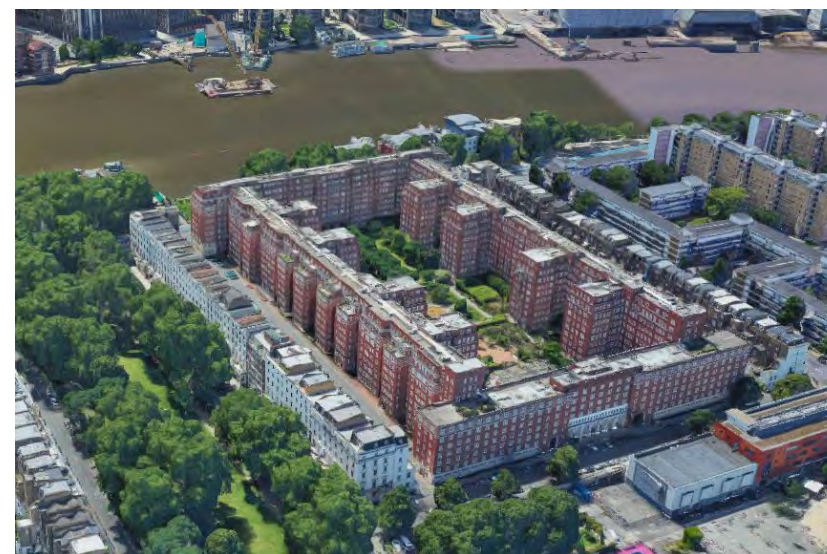
Figure 1.5.1 - Aerial image of site.
