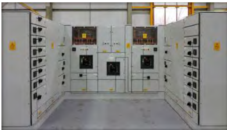
Figure 9.3.1: Typical U-shaped LV switchboard
