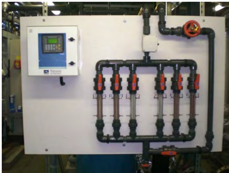
Figure 8.8.2 Typical Copper/ Silver Ionisation unit
