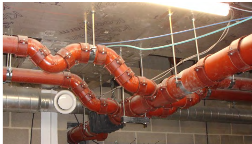
Figure 8.3.4 Typical lightweight cast iron drainage
