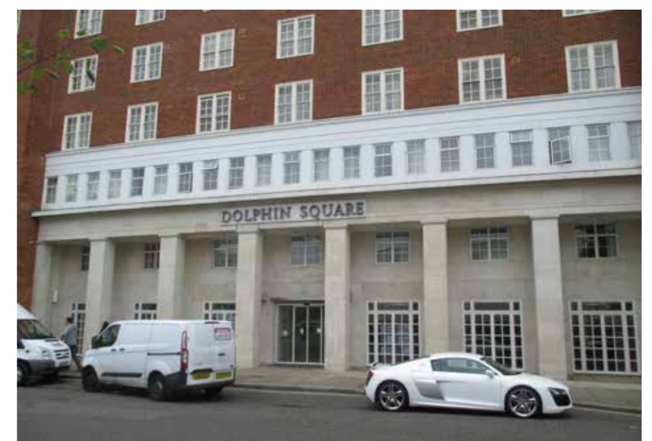
Fig 2.15: 2016 photograph showing the current Chichester Street entrance of Rodney House, with alterations carried out in 2006, i.e., the glazed elements removed and alterations to the ground floor windows.
