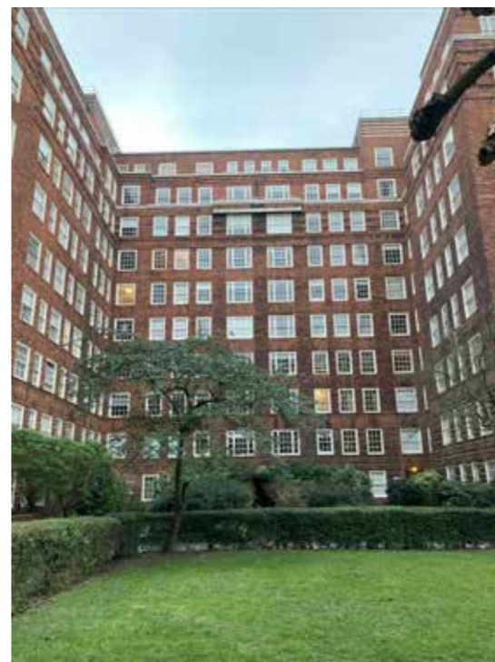
Fig. 3.13: Regular recess façade, one of eight
