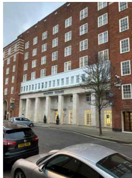
Fig. 3.7: The entrance colonnade
