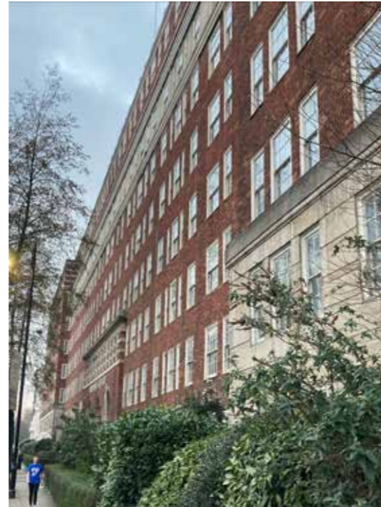
Fig. 3.10: Grosvenor Road façade
