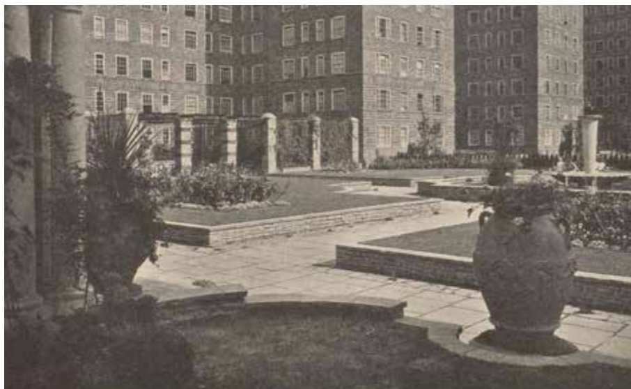
Fig 2.16: View from the pavilion towards the gardens from The Builder journal of 1937 (RIBA Library).
