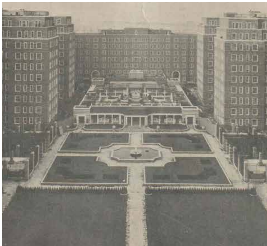
Fig 2.11: View of Dolphin Square's internal courtyard with, at the centre of the image, the south frontage of Rodney House and the pavilion with the Spanish and Mexican garden on its roof (published in the Architect and Building News journal of 1938, RIBA Library).
