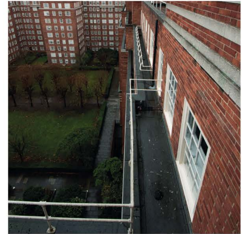
Roof setbacks - With guard
