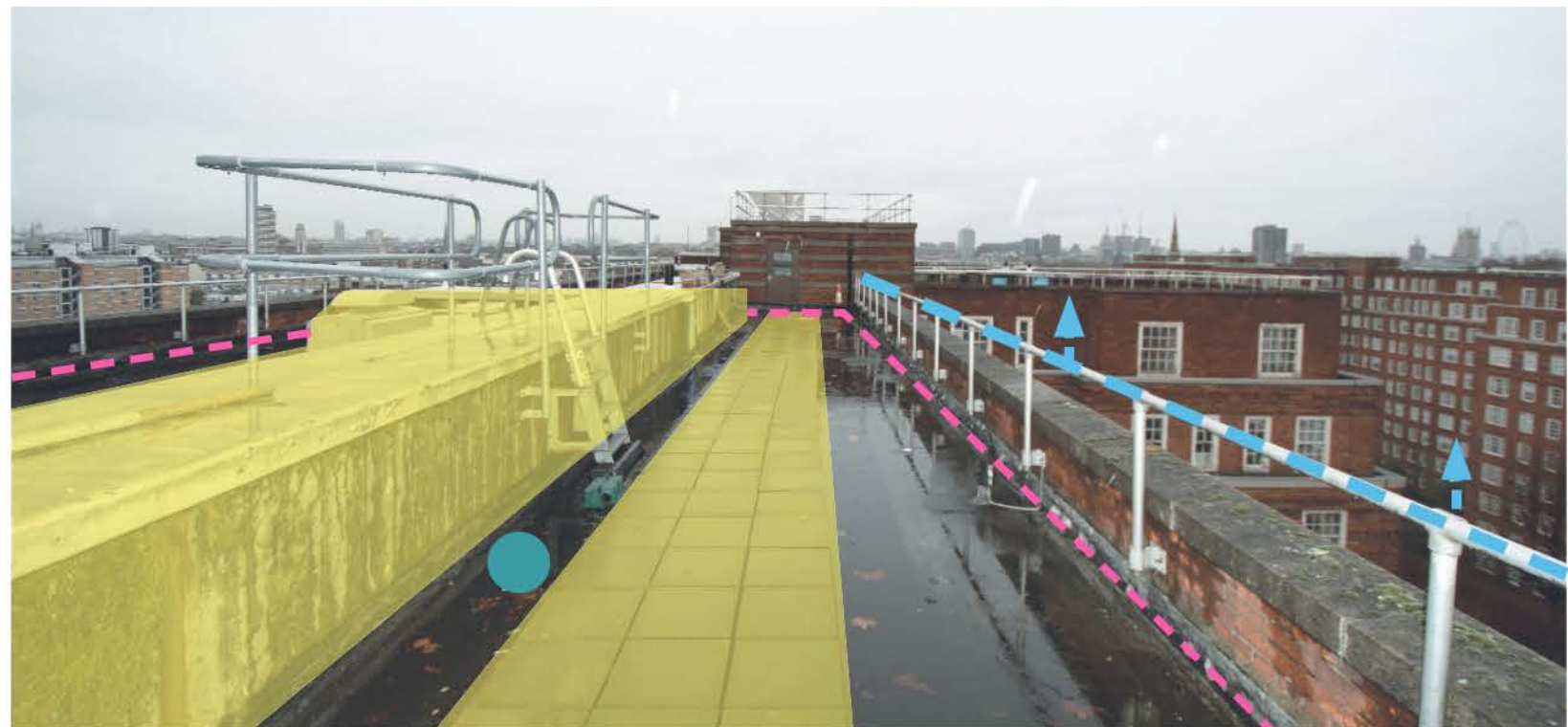
Typical roof - Intervention opportunities
