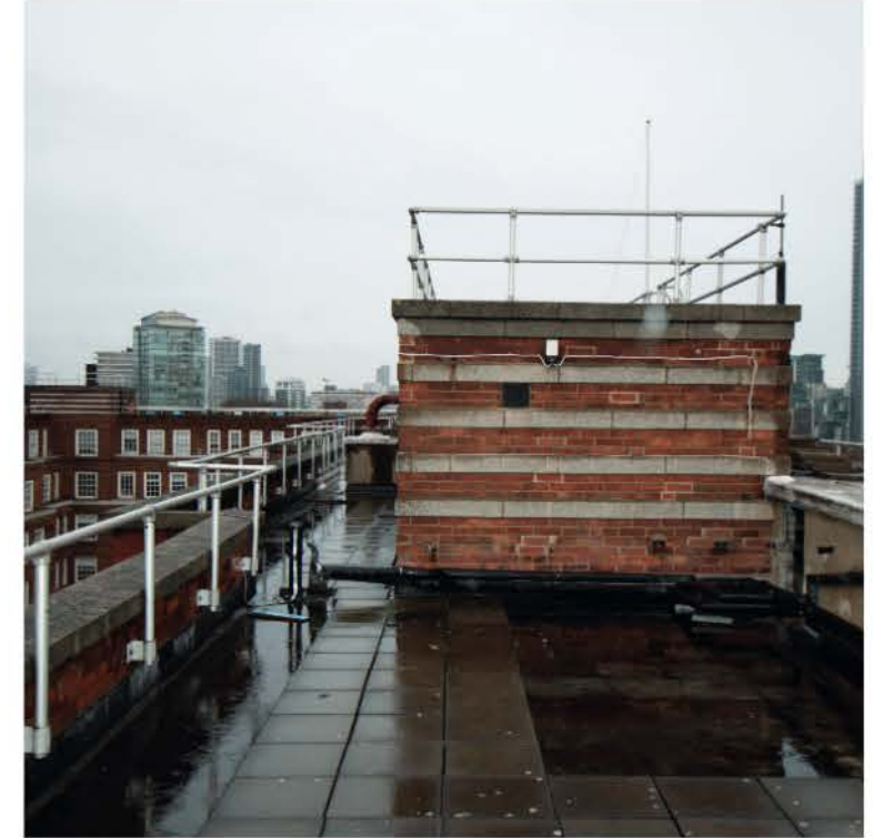
Typical roof environment
