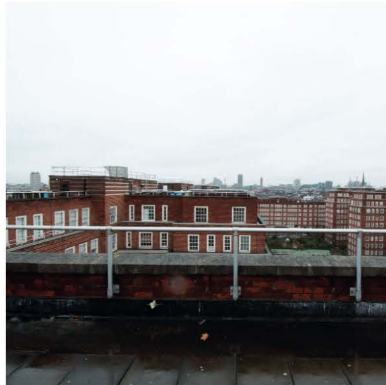
Typical roof environment - Parameter guarding
