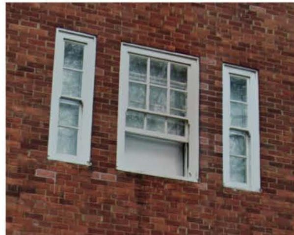
Existing constraint - Limited brickwork between windows
