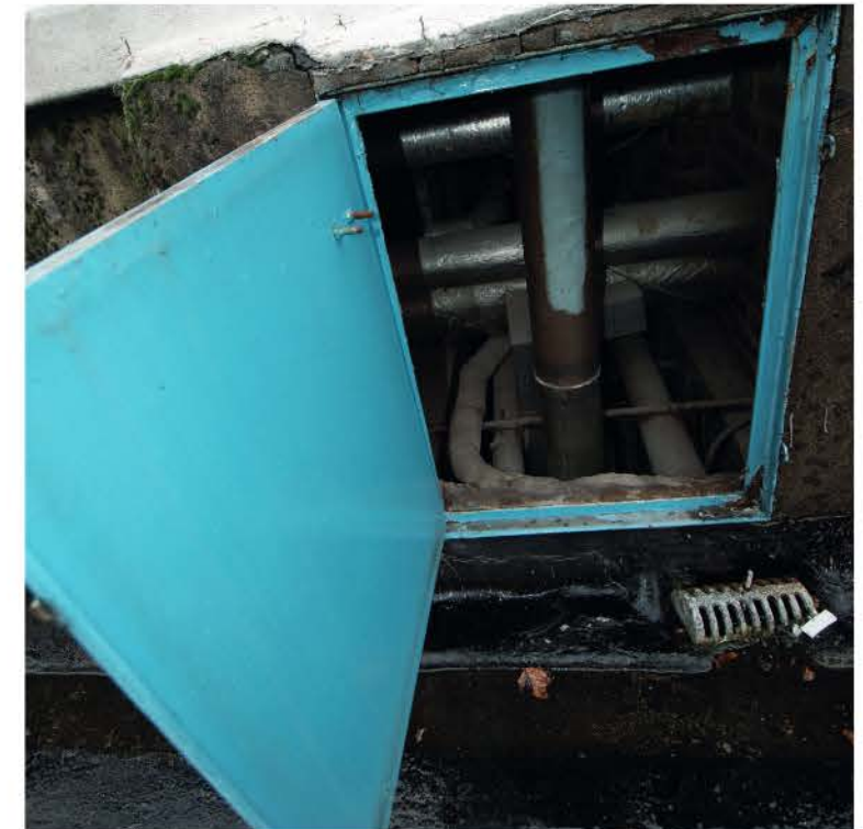
Typical roof environment - Services compartments
