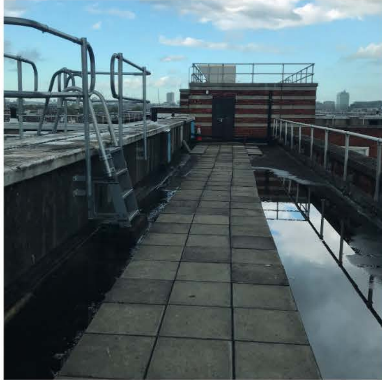
Typical roof environment
