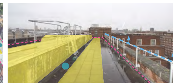
Typical roof Intervention opportunities
