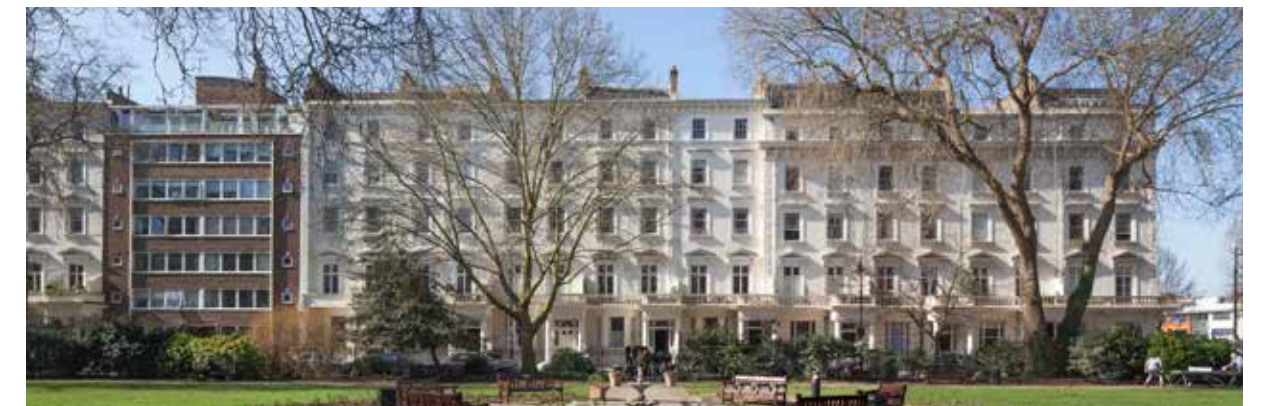
Fig. 6.3: View of Dolphin Square from St. George’s Square above the listed terrace
