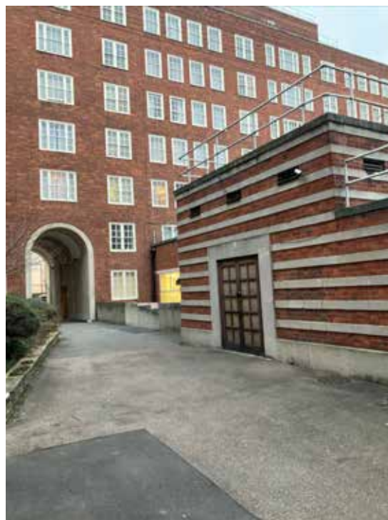
Fig. 3.18: Arched entrance from Chichester Street and north-west corner of amenity block
