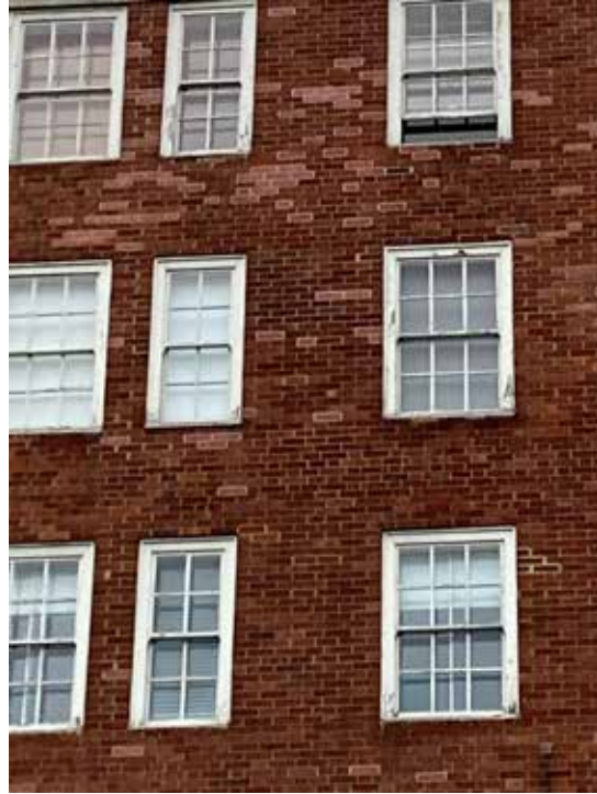
Fig. 3.21: Brick repairs post war damage
