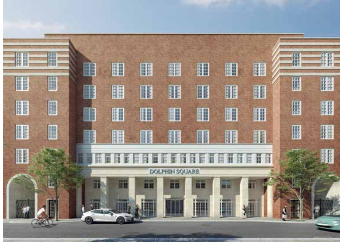
Fig. 5.1: Chichester Street Portico - Existing
