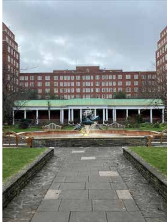
Fig. 3.15: Colonnade pavilion to south of amenity block
