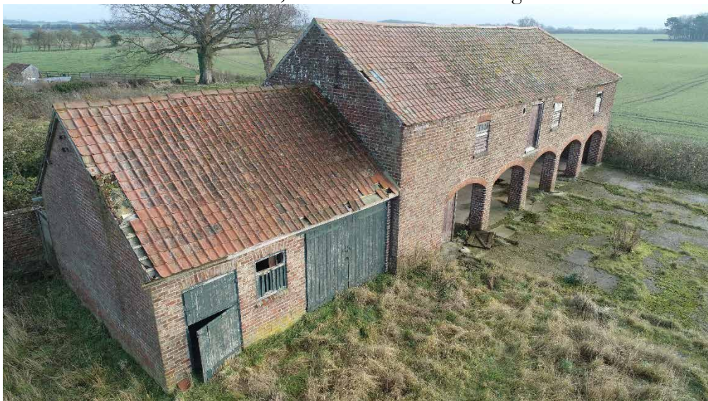
Plate 4 – Plot 2, west elevation and north gables.
