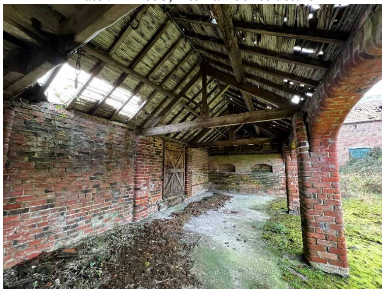
Plate 9 – Plot 3, internal roof structure.
