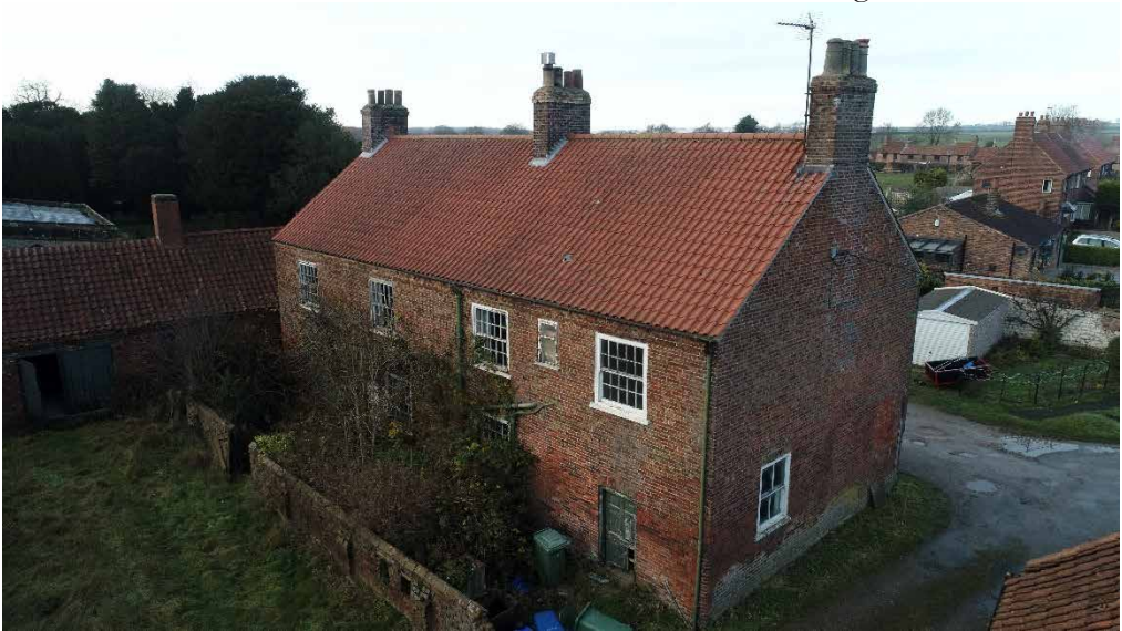
Plate 22 – Farm house, south elevation and east gable.
