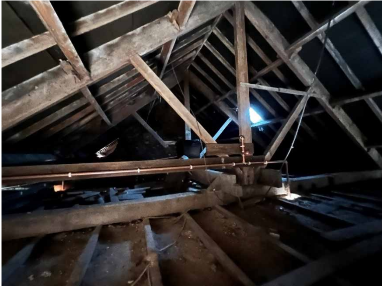
Plate 23 – Farm house, internal roof void.
