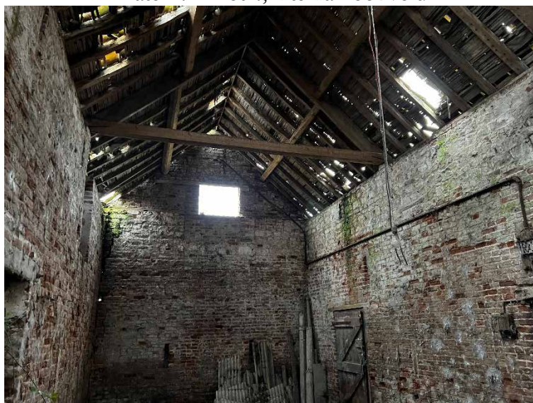
Plate 14 – Plot 4, internal roof void
