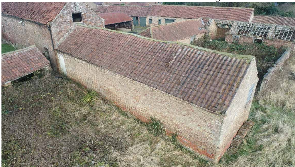
Plate 13 – Plot 4, west elevation and south gables.
