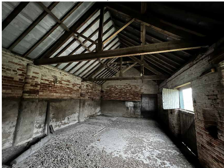
Plate 3 – Plot 1, internal roof void.
