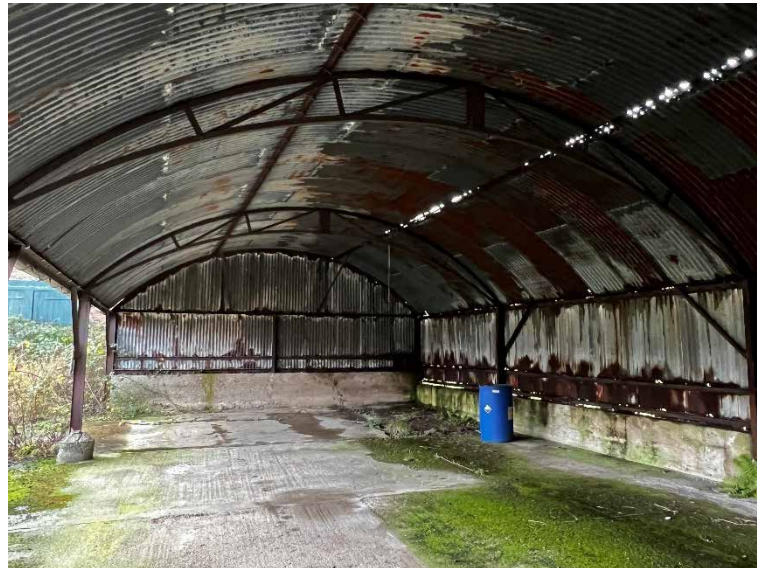
Plate 20 – Nissen hut internal roof structure.
