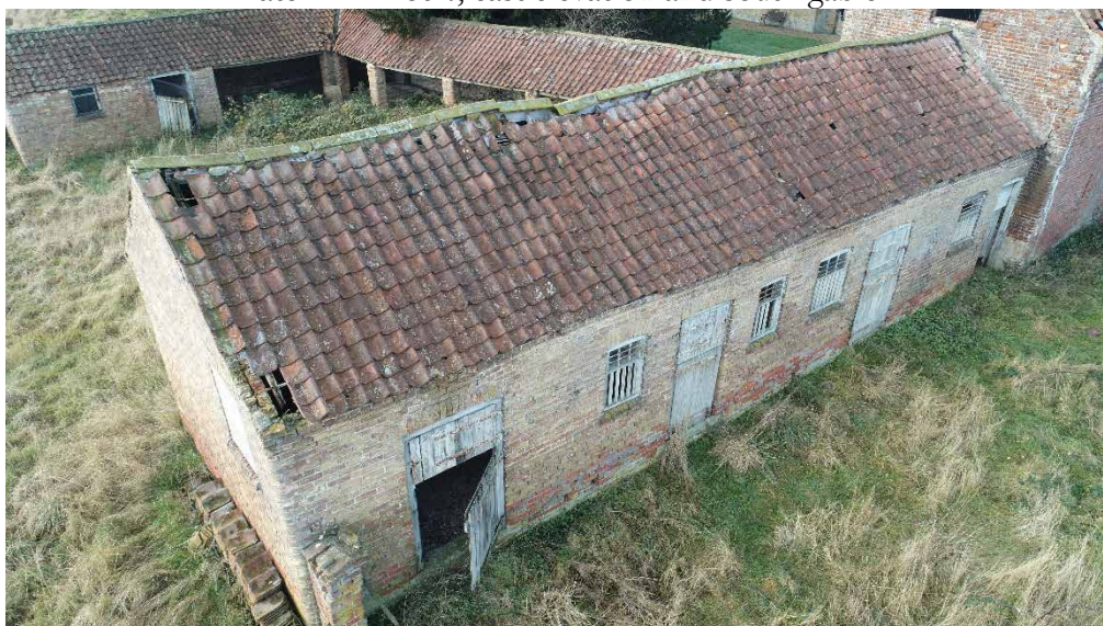
Plate 11 – Plot 4, east elevation and south gable.
