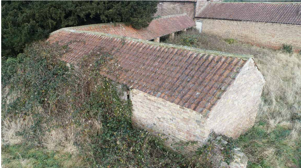
Plate 17 – Plot 5, east elevation and south gable.
