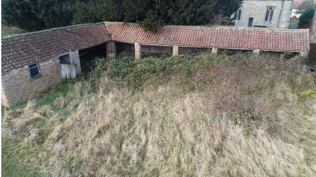
Plate 16 – Plot 5, south and east elevations.
