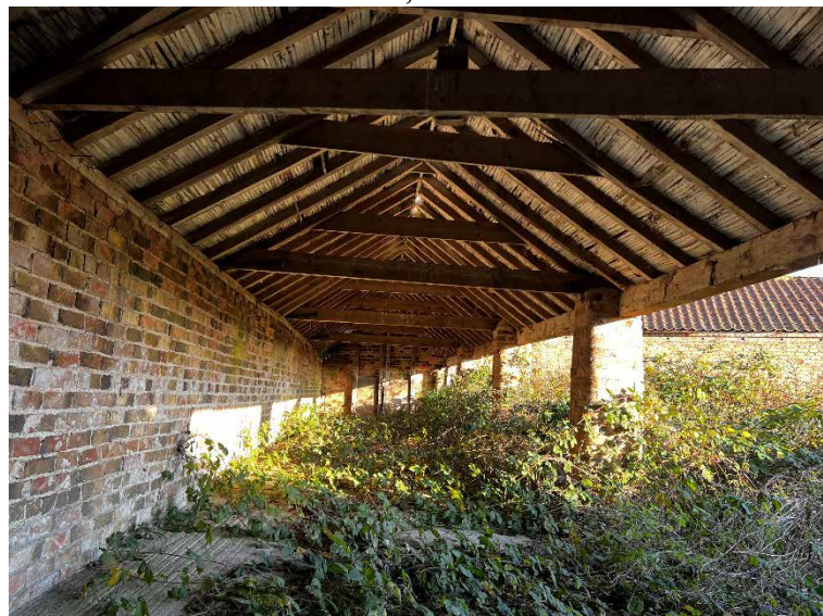
Plate 18 – Plot 6, internal roof void
