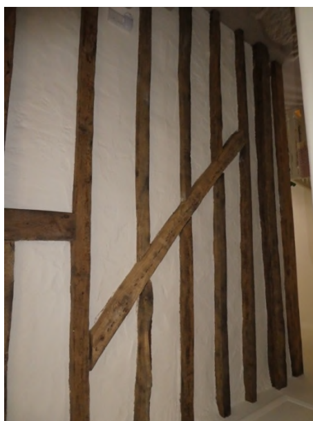
Figure 19: Stud partition in the passage to the rear wing
