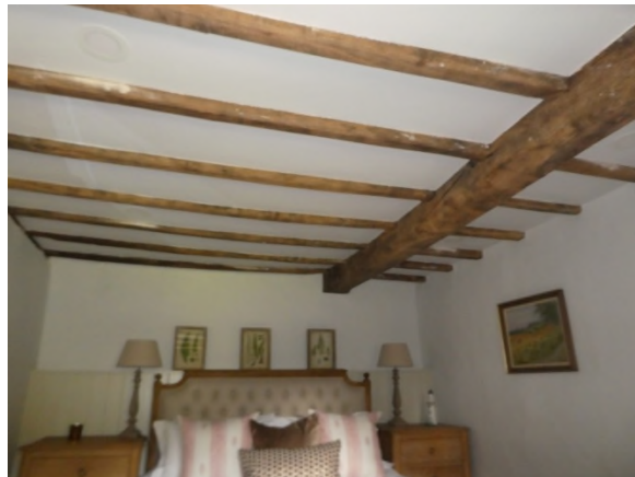
Figure 39: Transverse beam in the bedroom
