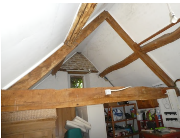
Figure 44: Butt purlin roof structure of the outbuilding
