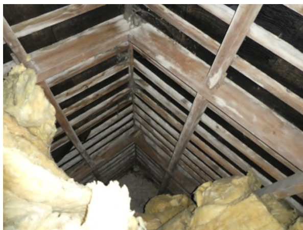
Figure 20: Replacement roof structure
