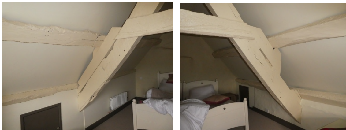
Figures 30 and 31: Roof structure in the attic bedroom
