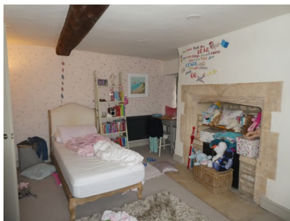
Figure 29: Transverse beam and stone fireplace in the first floor bedroom
