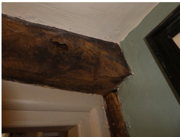
Figure 28: Ogee stop to the chamfered beam over the door to the W.C.
