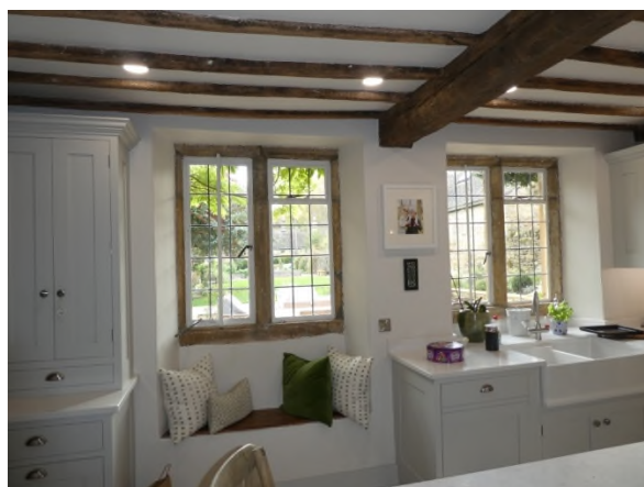
Figure 37: Chamfered mullion windows on the south-east side of the kitchen
