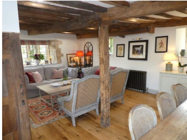
Figure 13: Timber post positioned under a scarf joint in the axial beams
