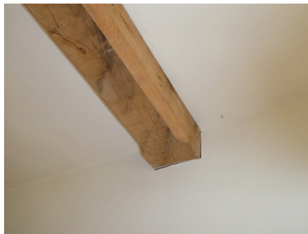
Figure 17: Later machine sawn beam in the bedroom
