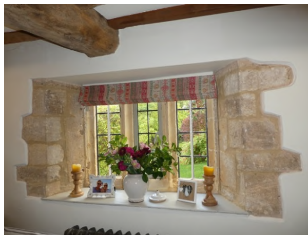
Figure 14: Axial beam with curved step stops and a 3-light window with hollow chamfered mullions on the south-east side of the ground floor
