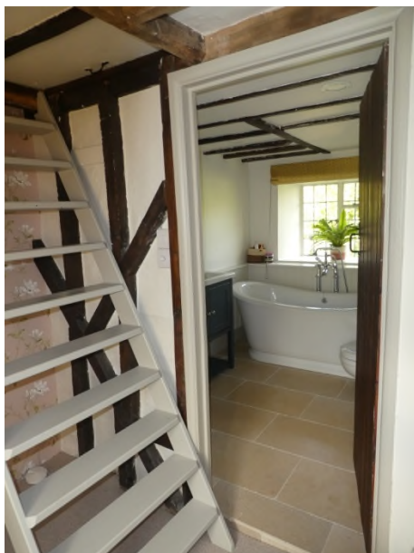
Figure 41: Stud partition to the bathroom on the first floor
