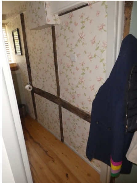
Figure 24: Timber framed partition in the W.C.
