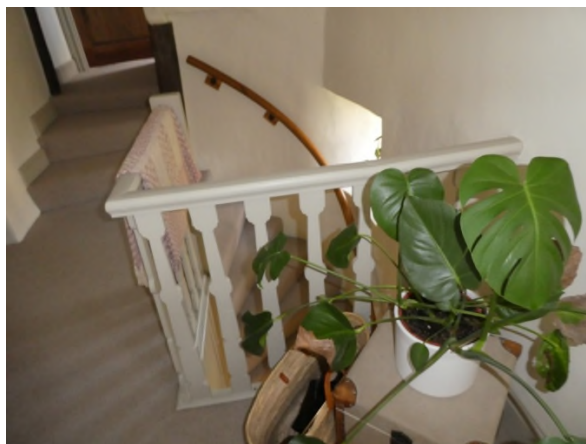
Figure 18: Splat balusters to the first floor balustrade
