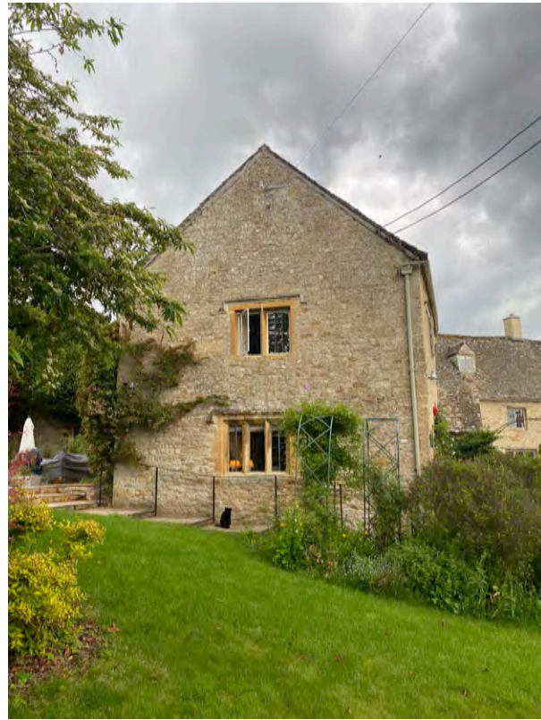
South eastern gable
