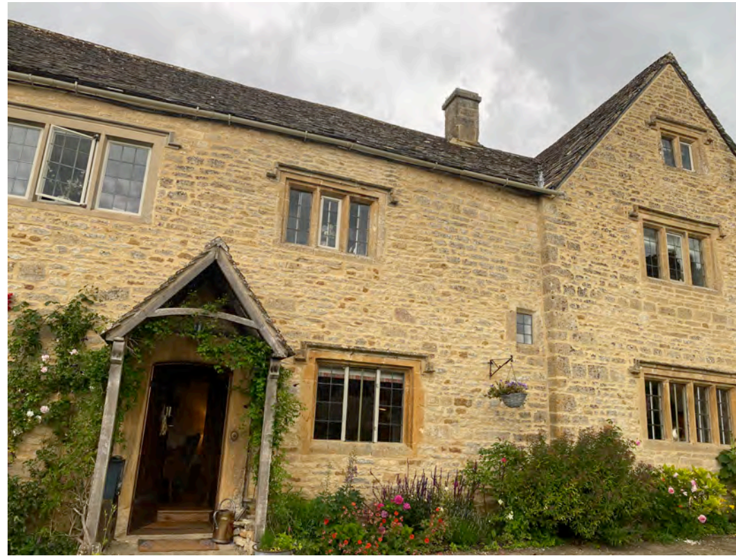
Frontage to road, main entrance
