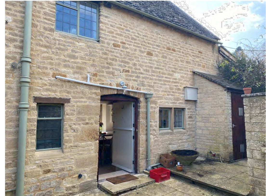
North western face of kitchen
