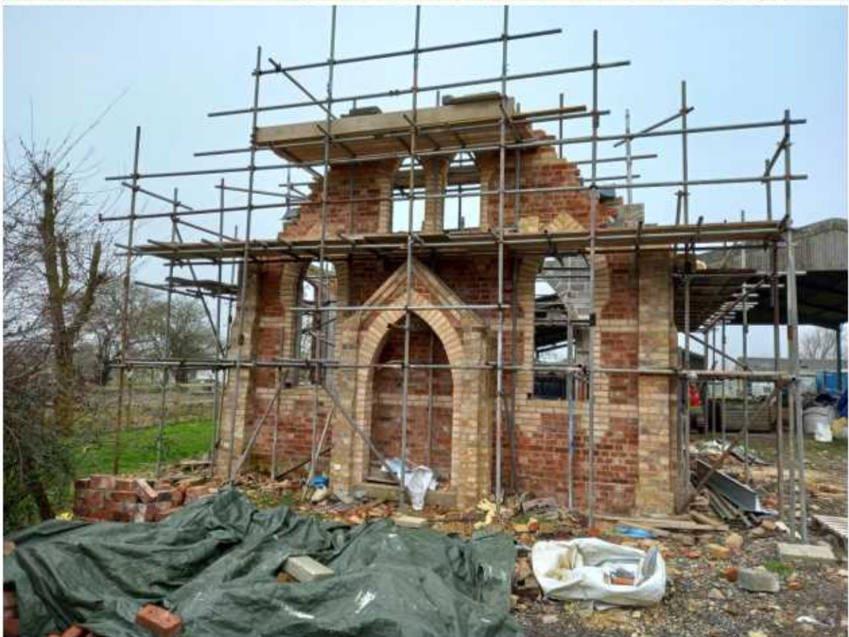
Figure 6: The current progress of the rebuilt structure.
