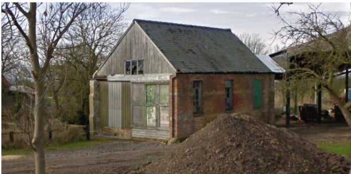
Figure 3: The original barn which was to be converted to a dwelling under Permitted Development.
