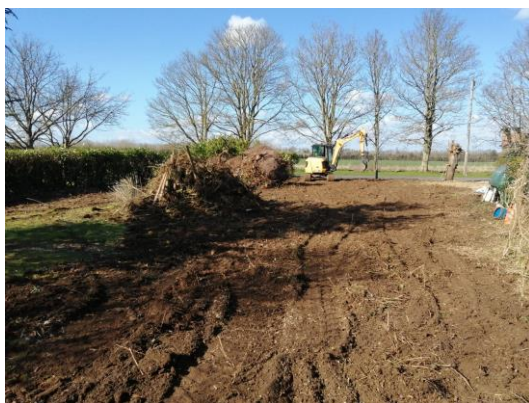
View Across Site towards Rostrop Road (North Facing)
