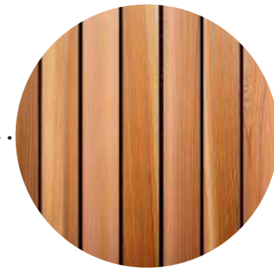
Vertical timber cladding
