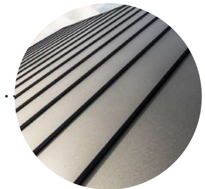
Profiled metal roof
