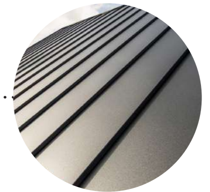
Profiled metal roof
