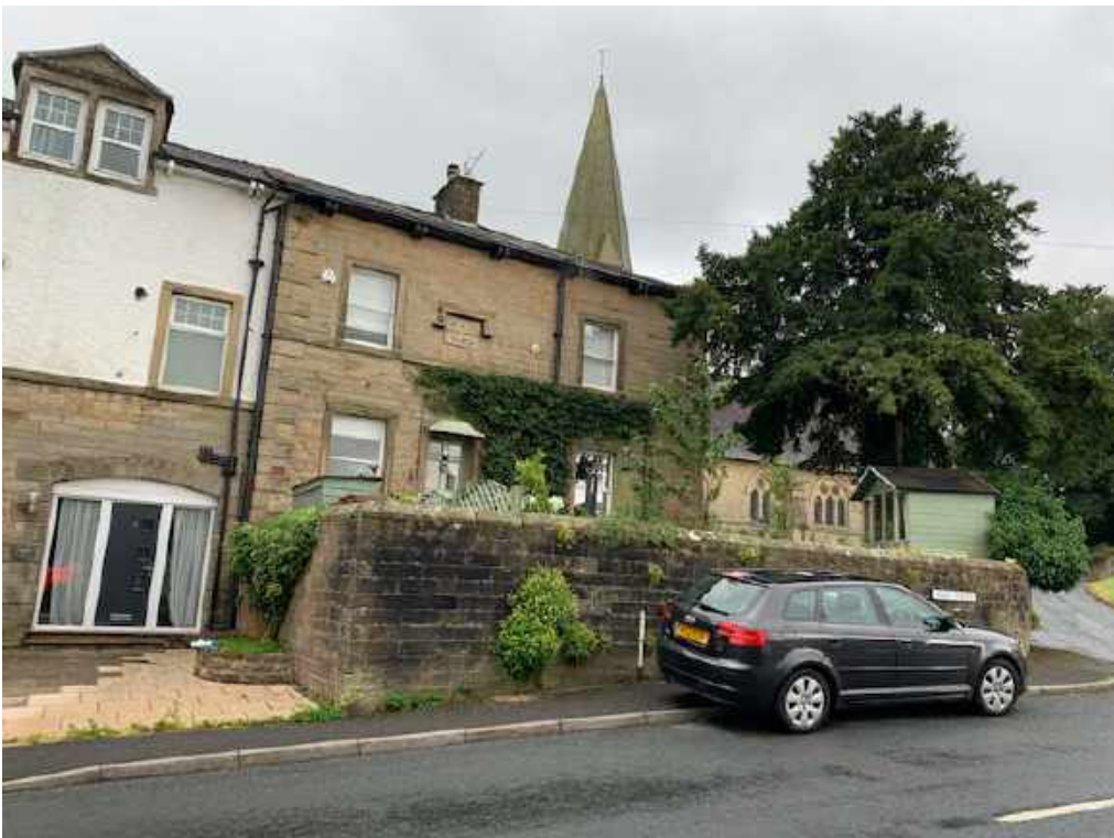
Existing front elevation – the view of the dwelling from High street
