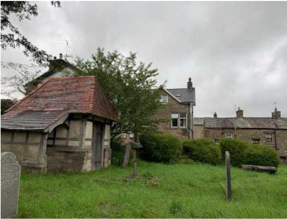
Existing rear elevation – the view of the dwelling from the Church graveyard
