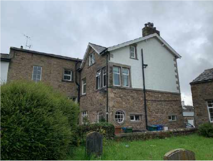
Figure 10 – view of dwelling from graveyard
