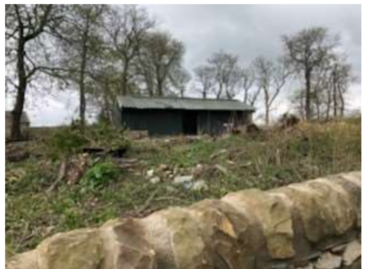
East elevation of shed from highway boundary
