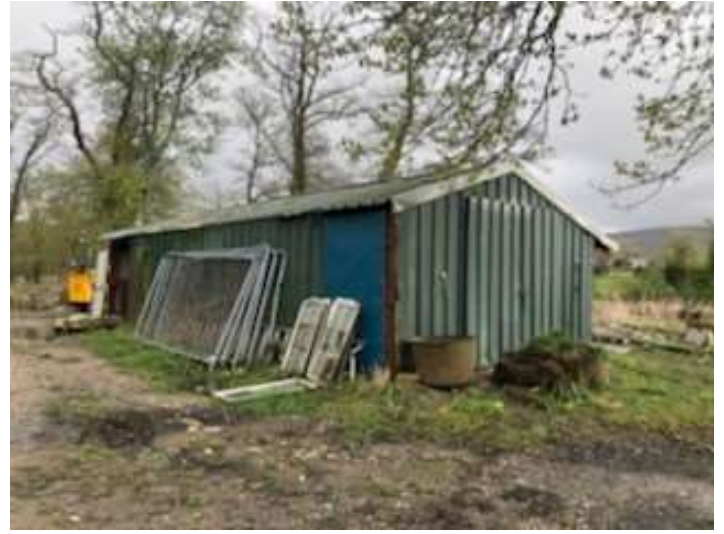
Shed from southwest
