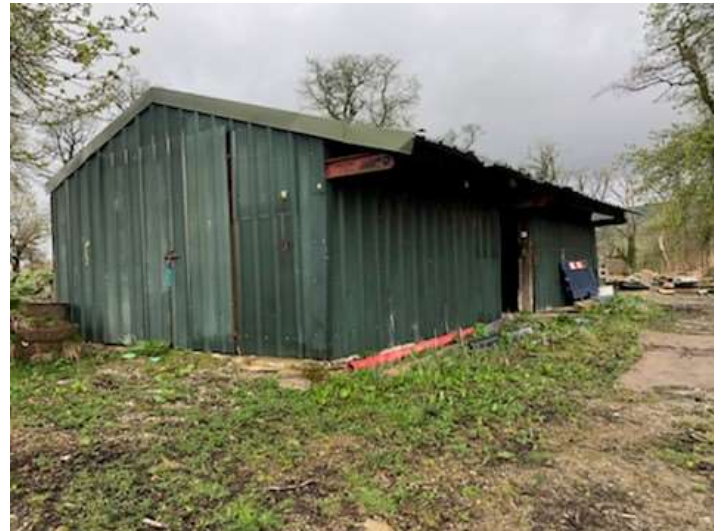
Shed from southeast
