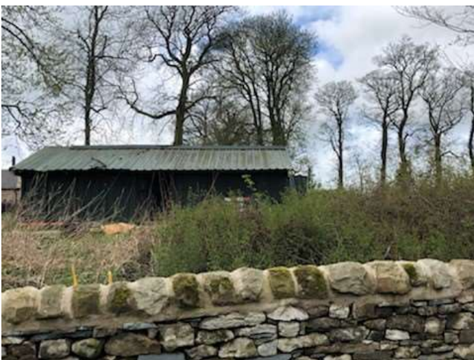
East elevation of shed from highway boundary
