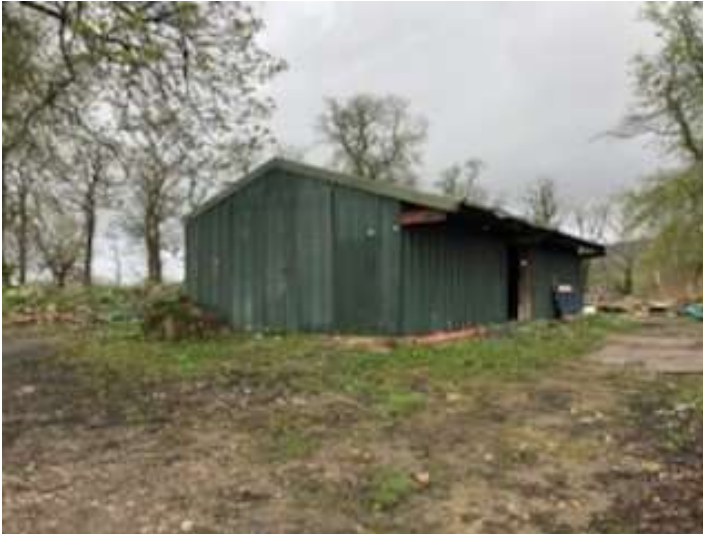
Approach to existing shed from southeast
